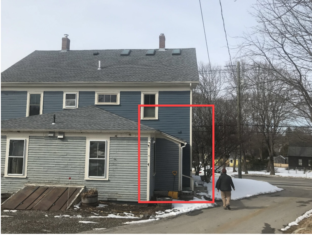
Figure 6: Current configuration of entrance to 978 South Street, overview.
