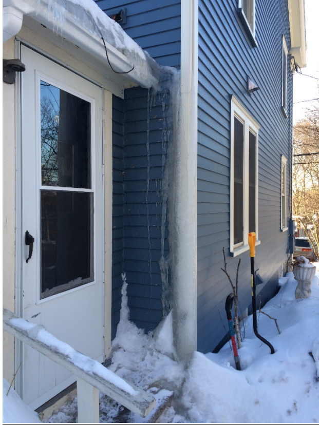
Figure 10: Example of ice build-up near 978 entry.
