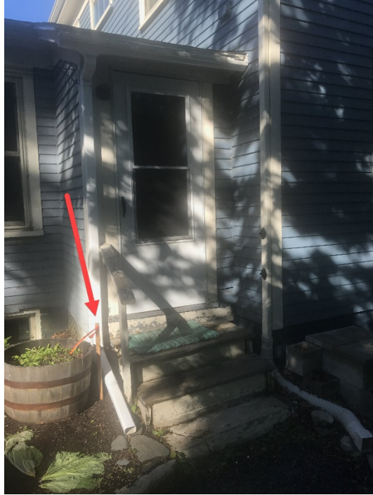
Figure 7: Current configuration of entrance to 978 South Street. Red arrow is drawing attention to boundary stake in image. Also shows current stairs extending beyond the property line.
