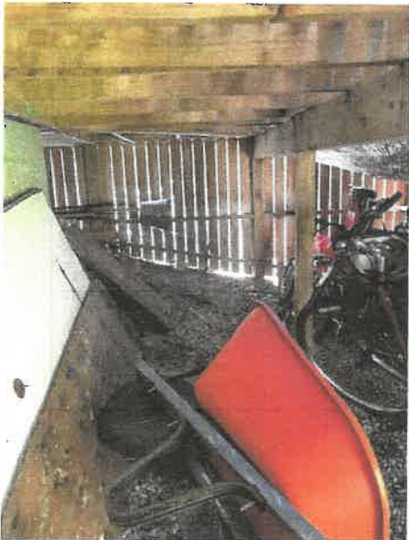
Under existing deck.
