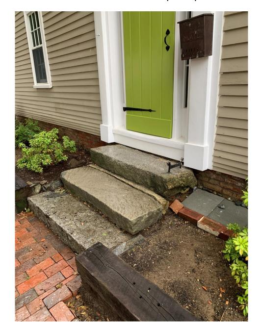
A new landing, 30" deep and the full width of the door frame from column to column, will allow us to better follow the building code and thus provide safer ingress and egress.
