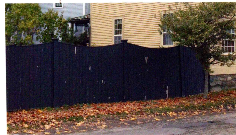
REPLACE FENCE IN KIND ALONG MARCY STREET, FROM ADDITION
