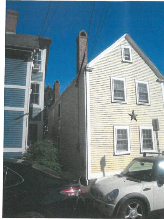
VIEW FROM SHEAFE STREET
