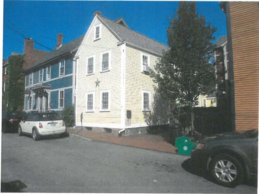
VIEW FROM SHEAFE STREET
