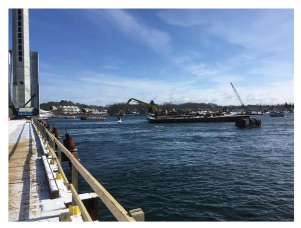
Photo 4: Example of a long-reach excavator operating from a barge during construction of the Sarah Mildred Long Bridge
