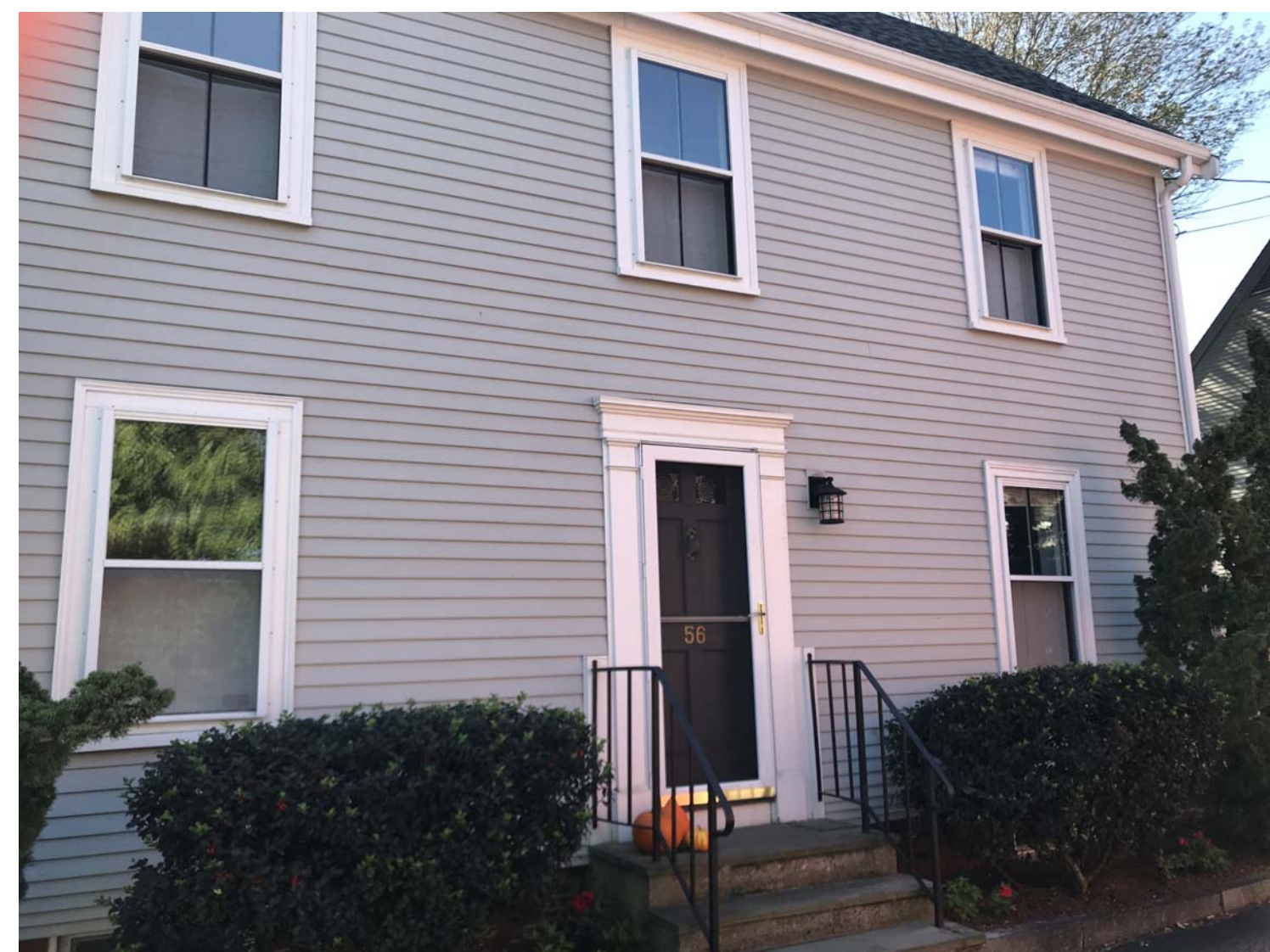
② Existing Conditions Photos 1/16" = 1'-0"
