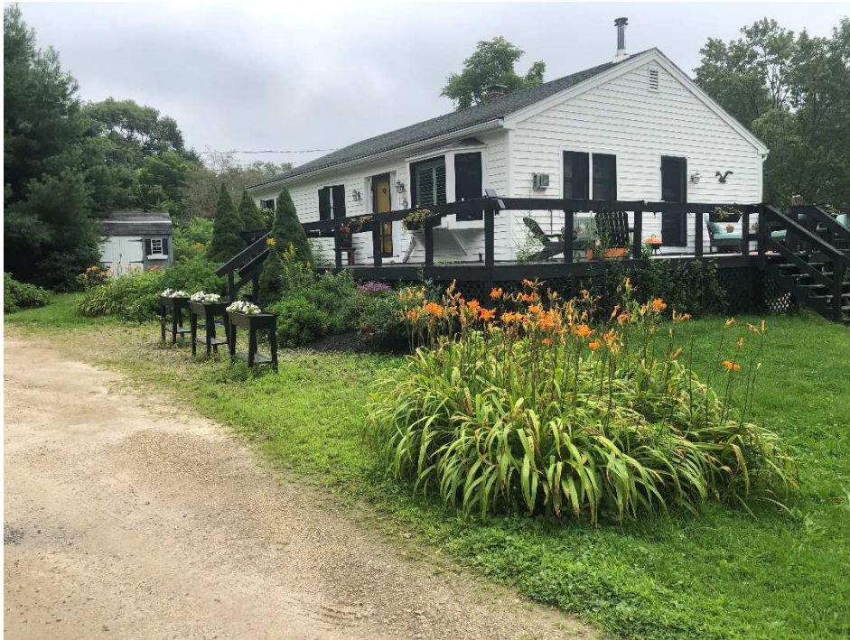
Photo 4: View of existing house looking towards the northeast. (August 9, 2021)
