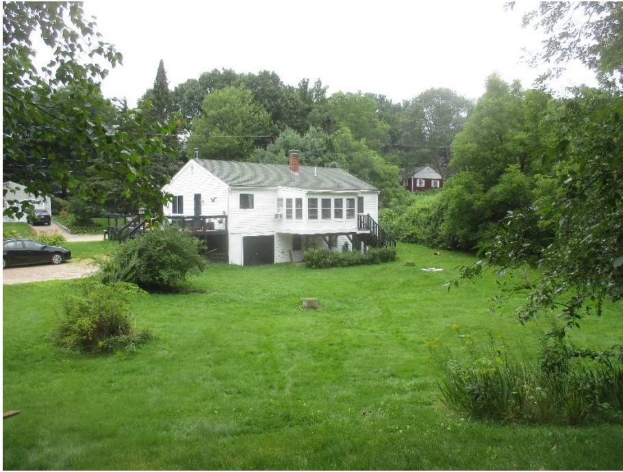
Photo 3: View of existing house looking towards the north. (August 9, 2021)
