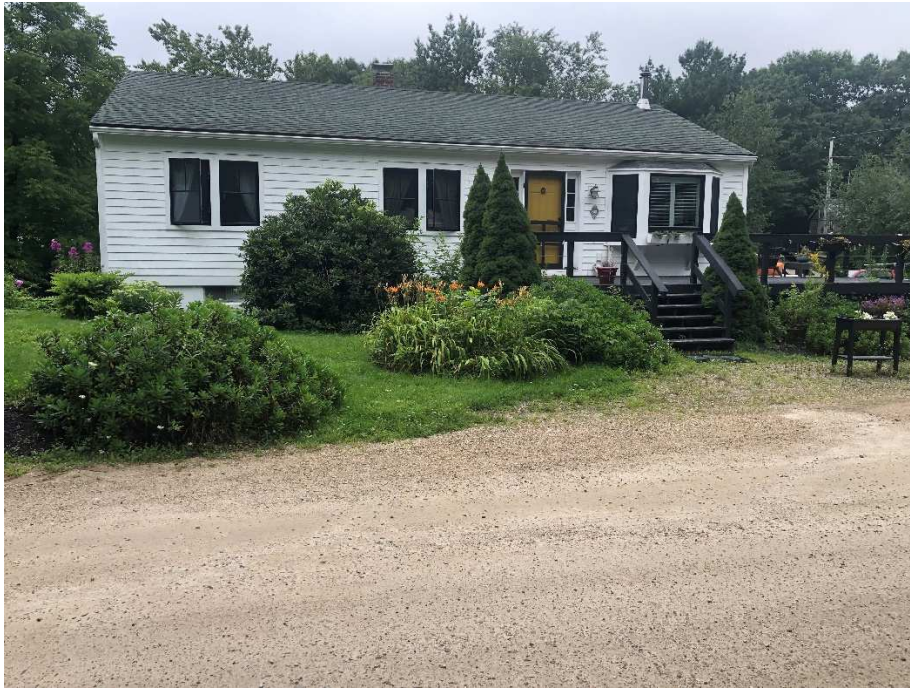
Photo 5: View of existing house looking to the southeast. (August 9, 2021)
