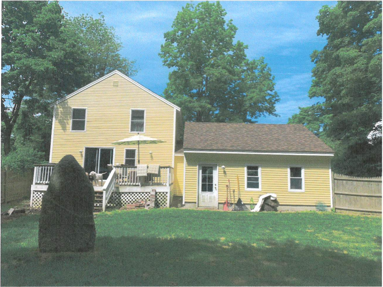
Rear View of House and Garage
