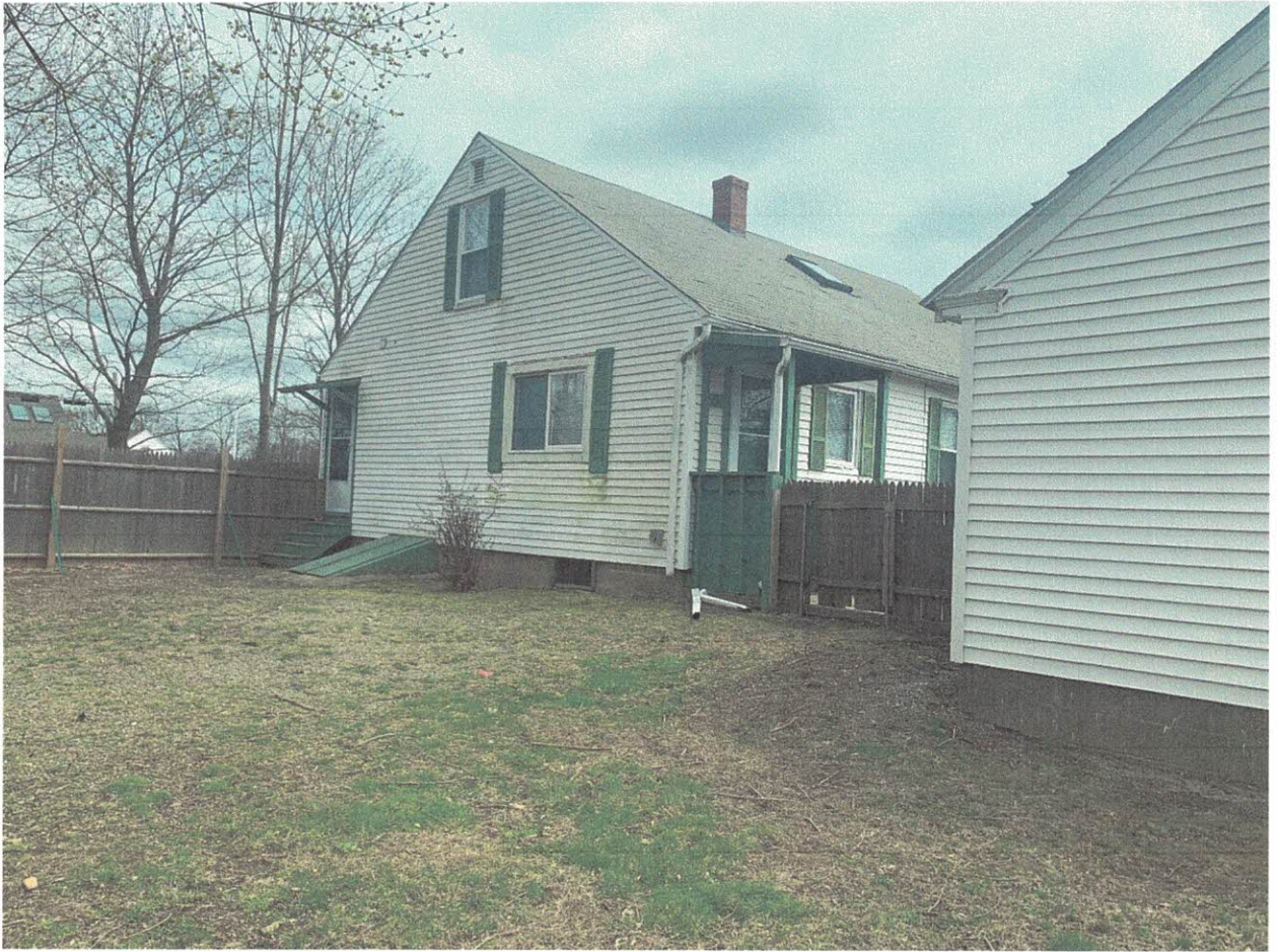
Rear Yard View of House and Detached Garage
