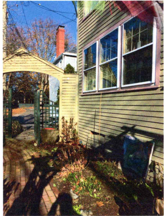
Entry Fence & Arch
