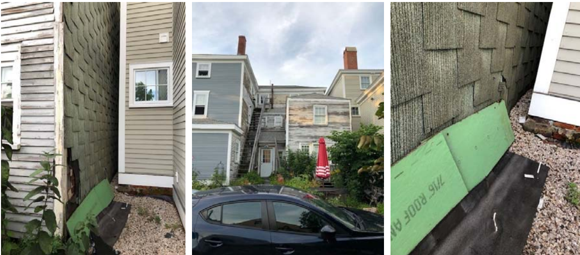
Middle photo shows the rear ell visibly leaning to the south. Outer photos show the area where the most significant sill rotting has occurred.
