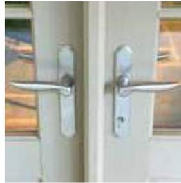
Lever handles for swinging doors are available in a variety of styles and finishes and make operation easier than doors with knobs.
