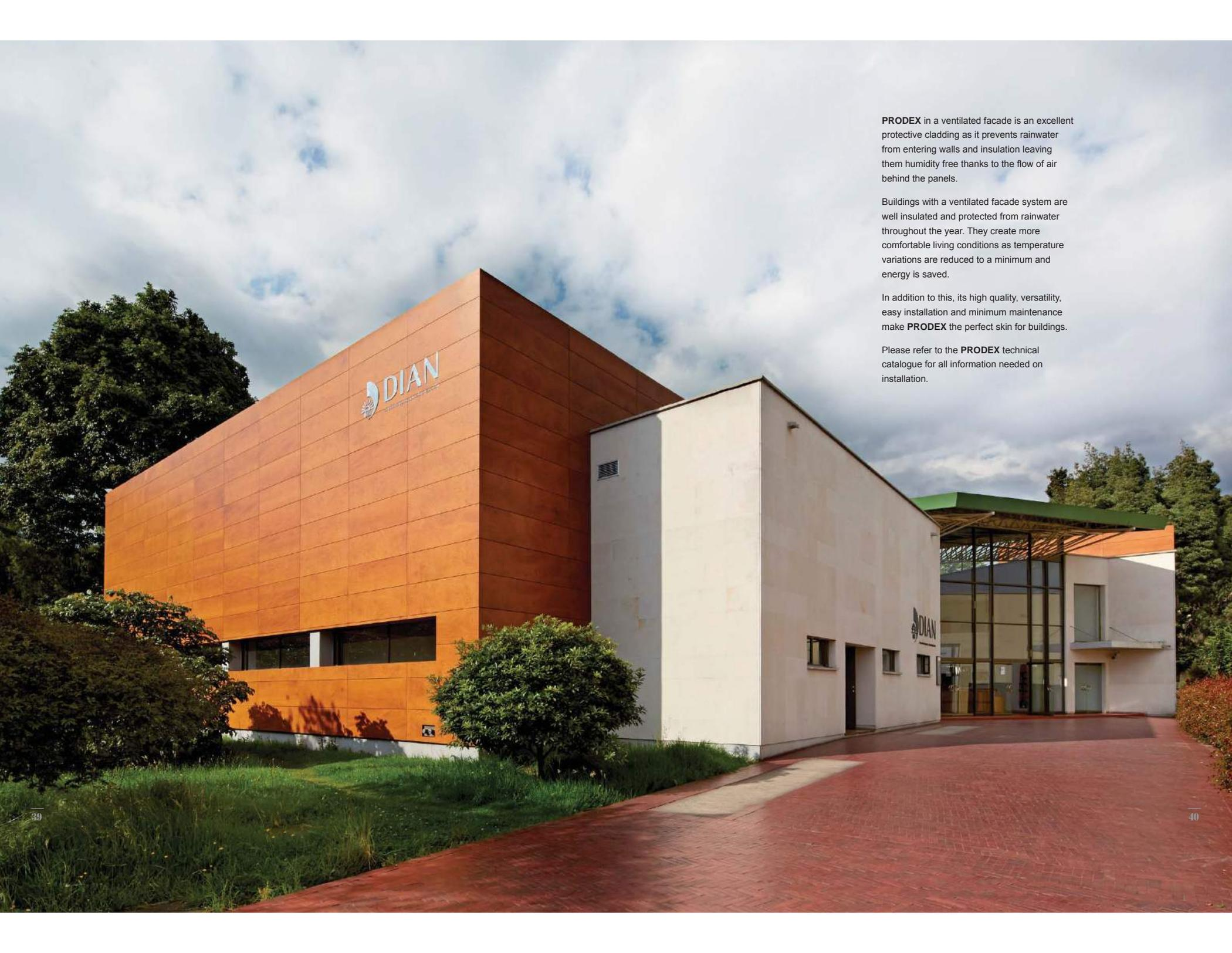
**PRODEX** in a ventilated facade is an excellent protective cladding as it prevents rainwater from entering walls and insulation leaving them humidity free thanks to the flow of air behind the panels.
