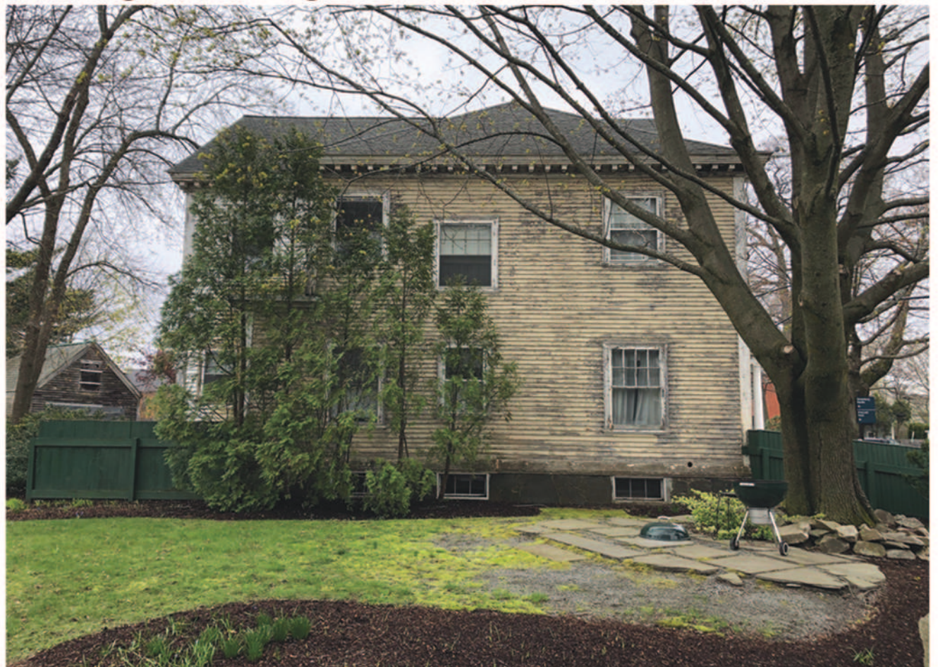
Existing Photo: Left Elevation
