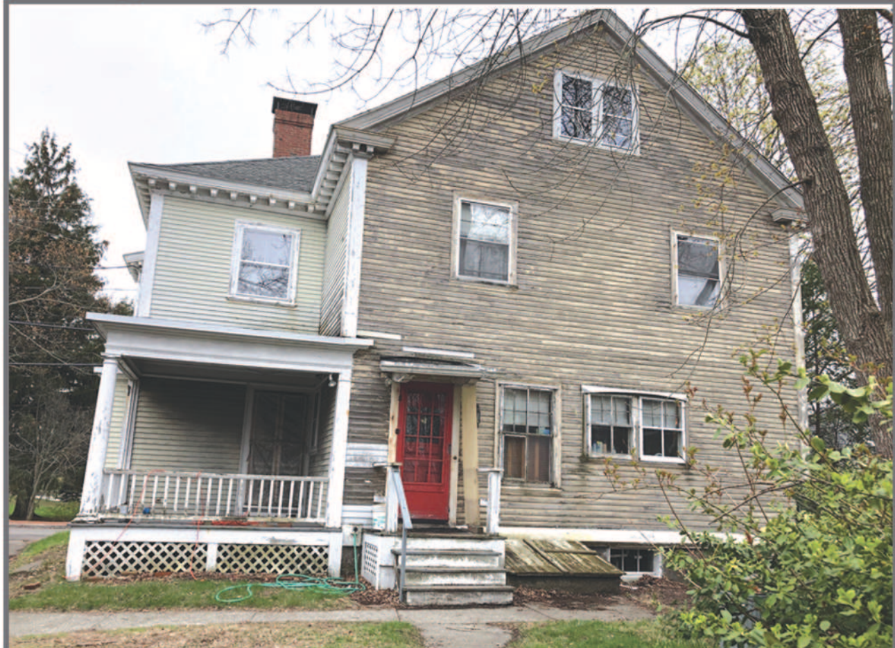
Existing Photo: Back Elevation
