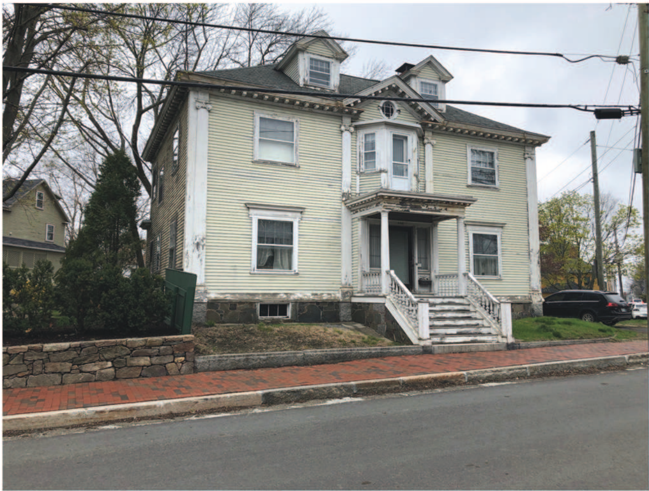
Existing Photo: Front Elevation
