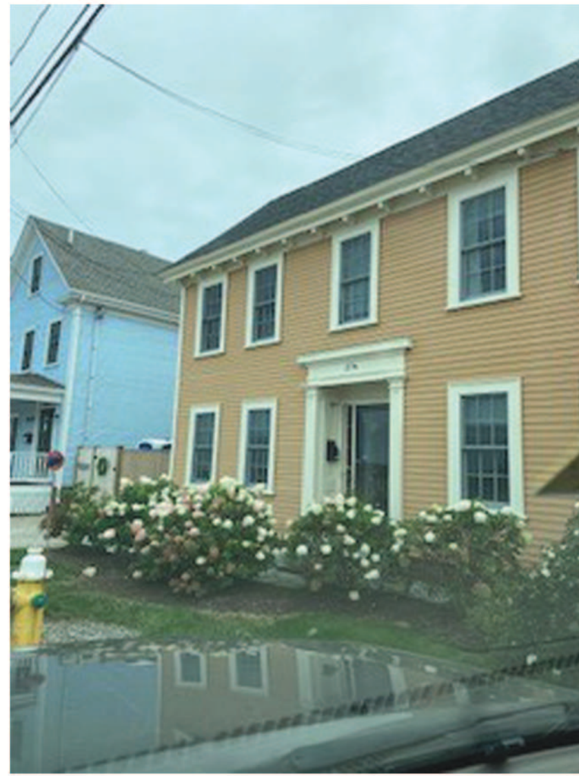
274 New Castle Ave: Approved window replacement
