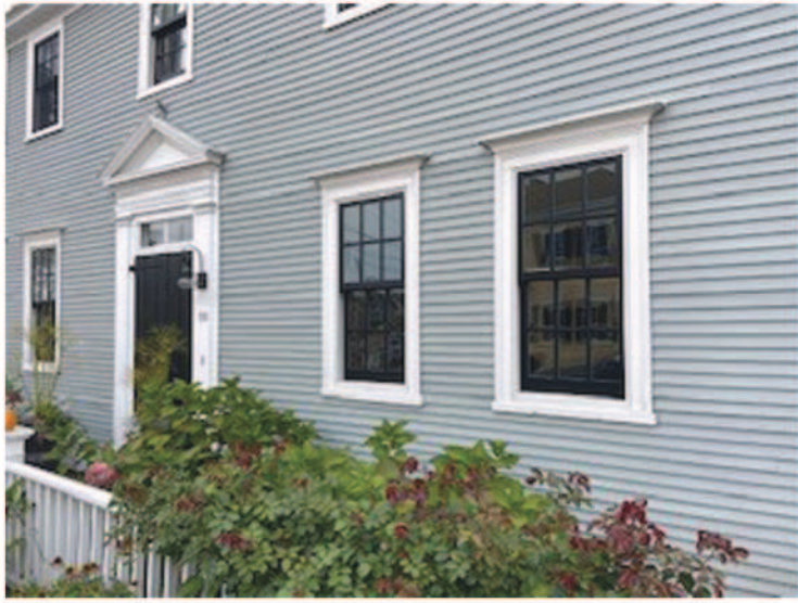
28 South Street: Approved window replacement
