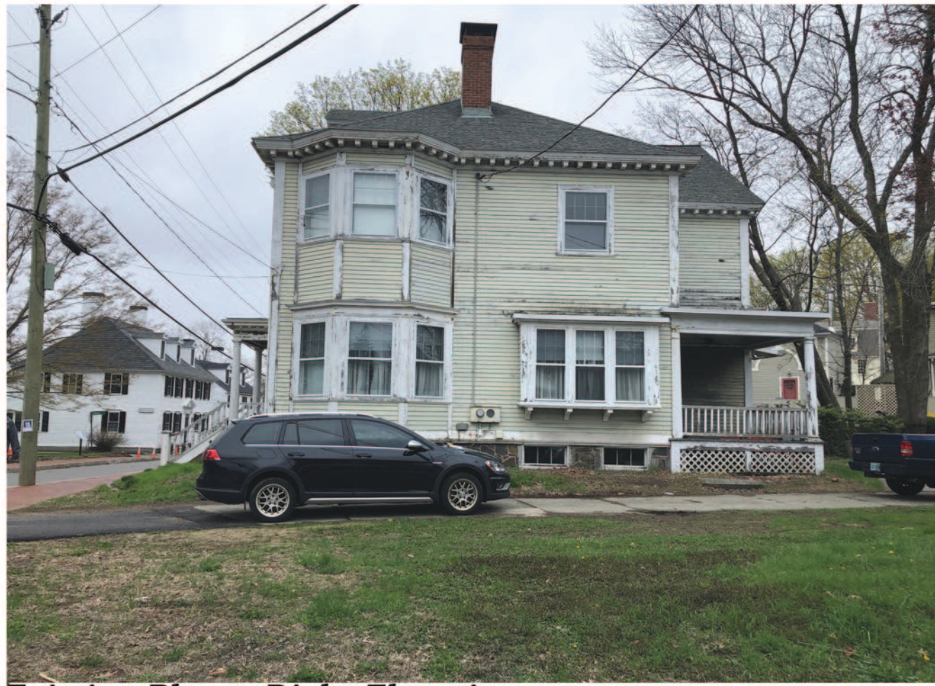
Existing Photo: Right Elevation
