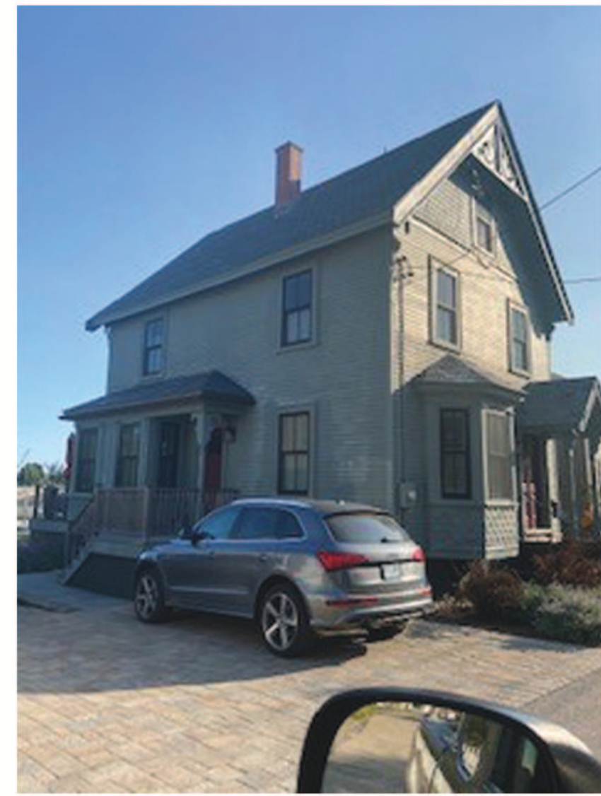
Salter Street: Approved window replacement in same style and manufacturer as proposed.
