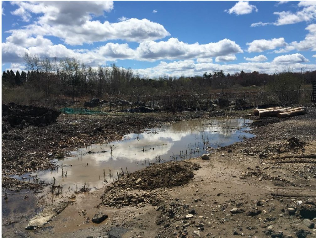
Photograph No. 9: Looking northerly at Wetland 6 (treatment swale).
