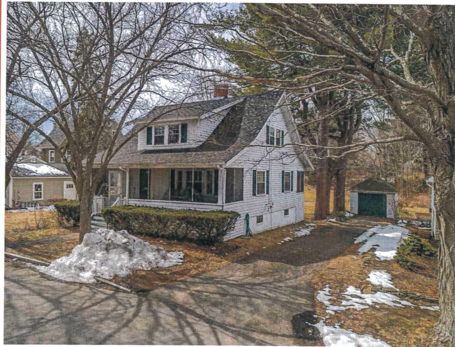
EAST FACADE FROM STREET
