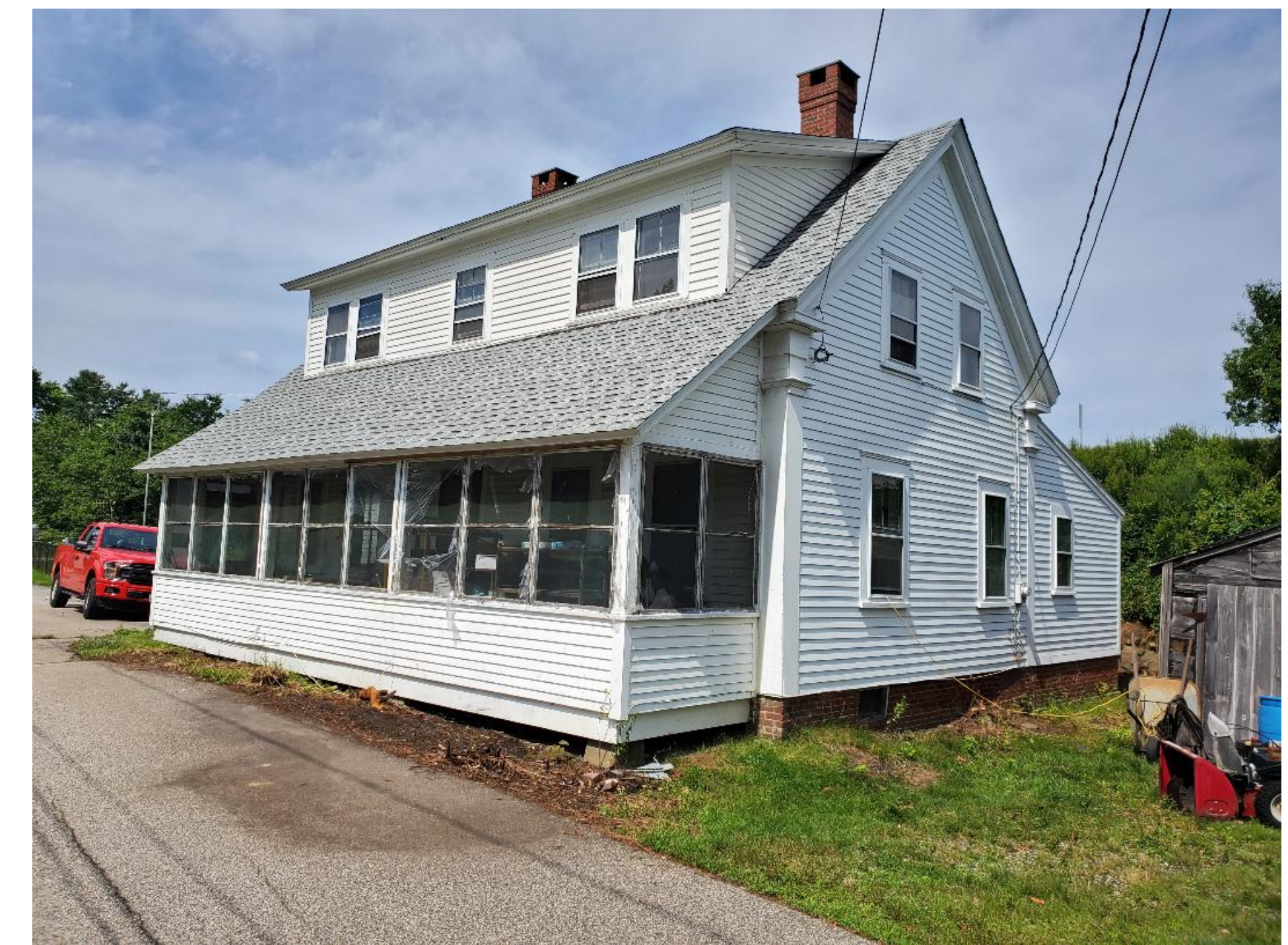
PHOTO- LOOKING AT NORTHWEST CORNER
