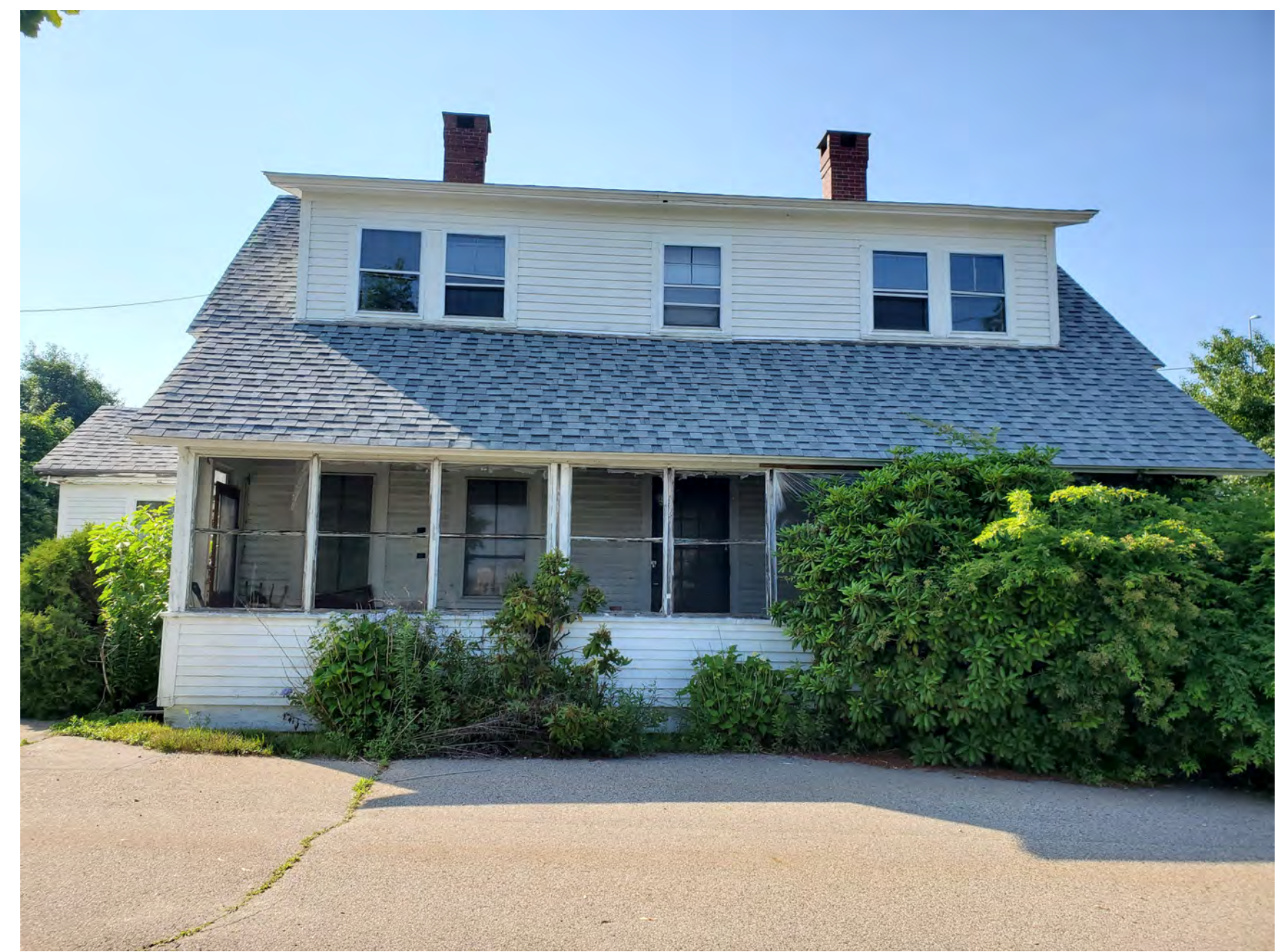
PHOTO- EAST ELEVATION
