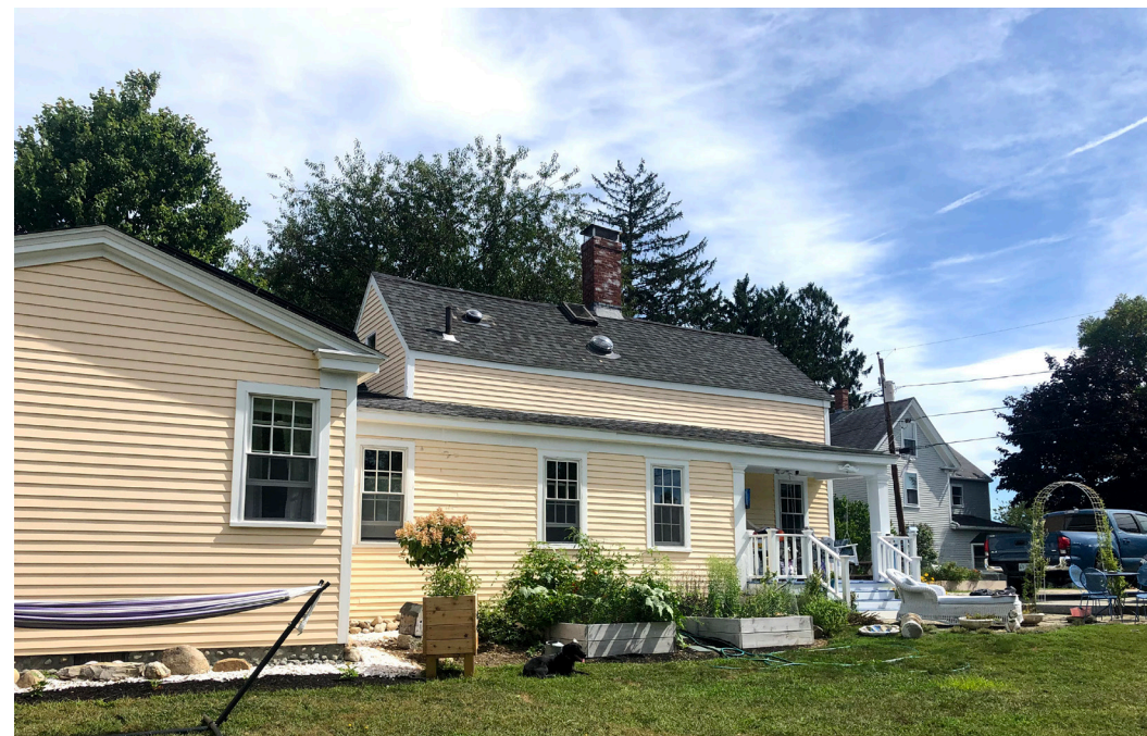
4 SOUTH EAST CORNER FROM YARD
