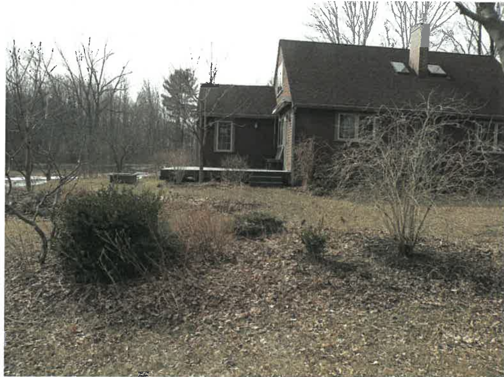
3. Looking west at the deck where the addition is proposed. The temporary impacts will start on the other side of this landscape bed.
