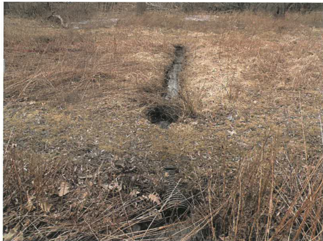
6. This is a view of one of the culverts to be removed.
