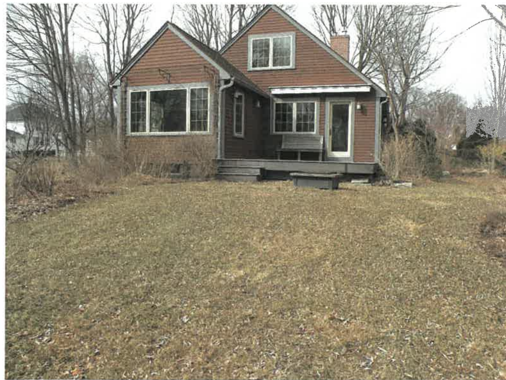
4. Looking north at the deck where the addition will go and the lawn area where the patio will go in front of the addition.
