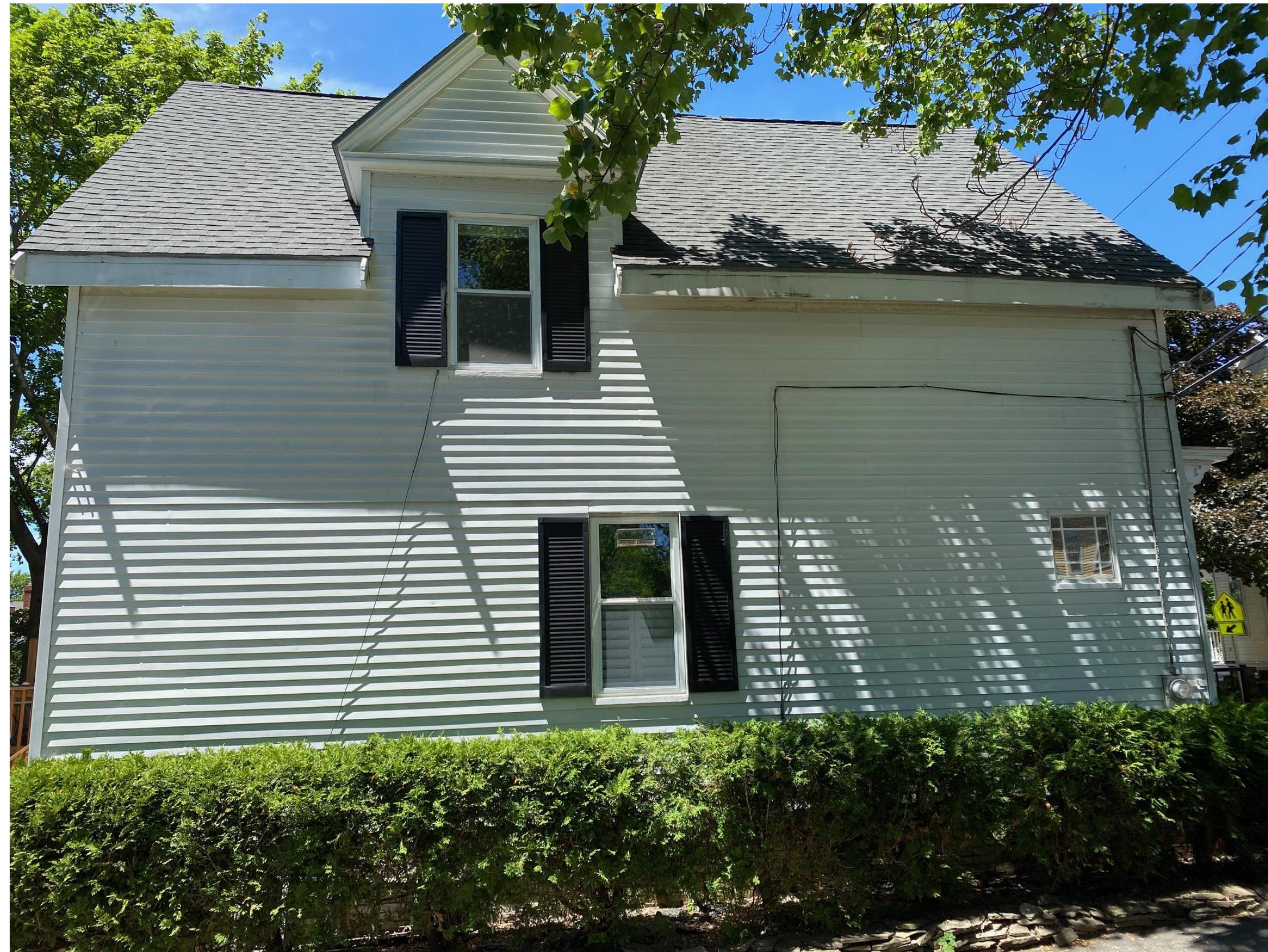
WEST ELEVATION PHOTO | SIDEVIEW
