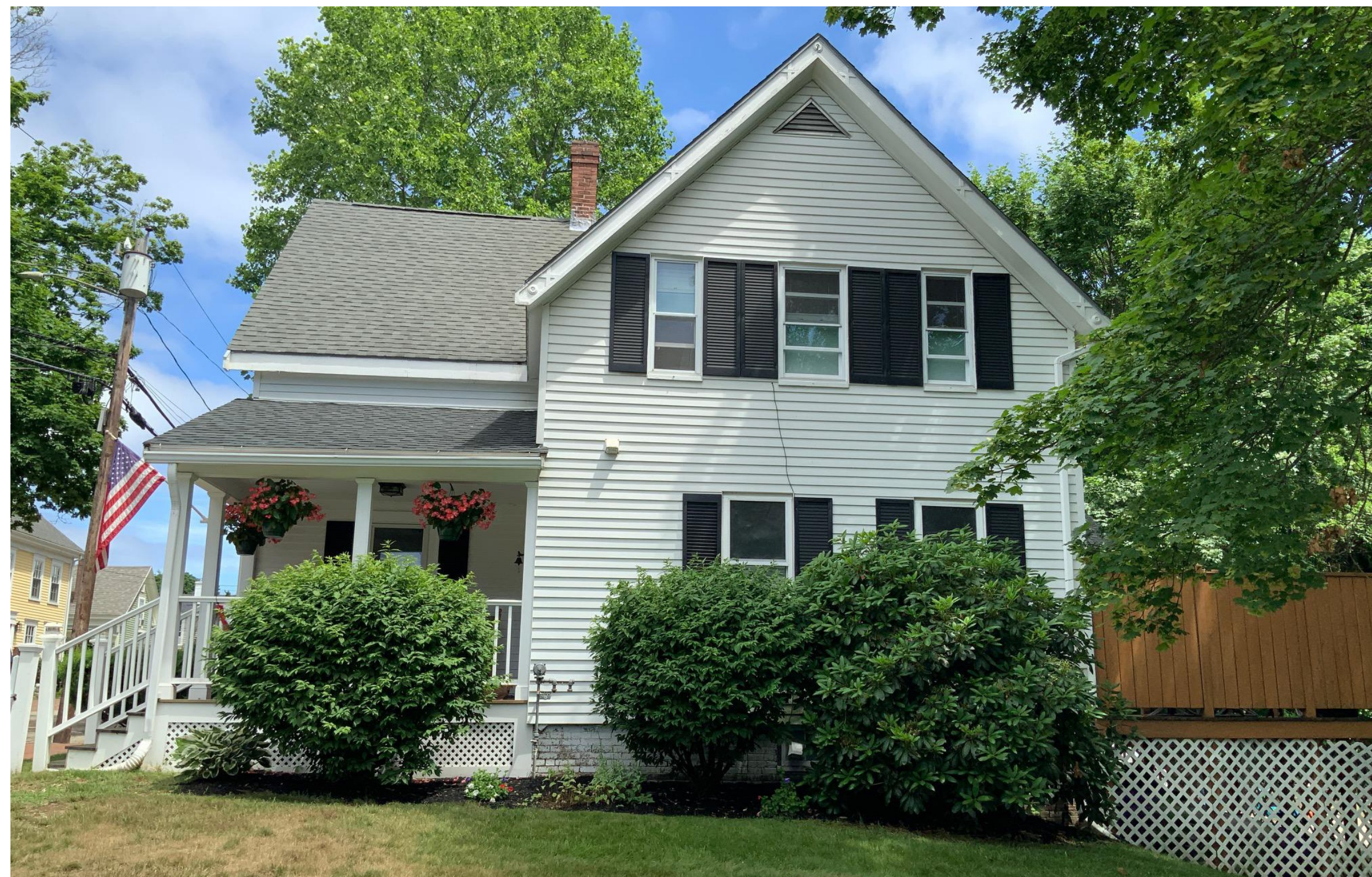
EAST ELEVATION PHOTO | SIDEVIEW
