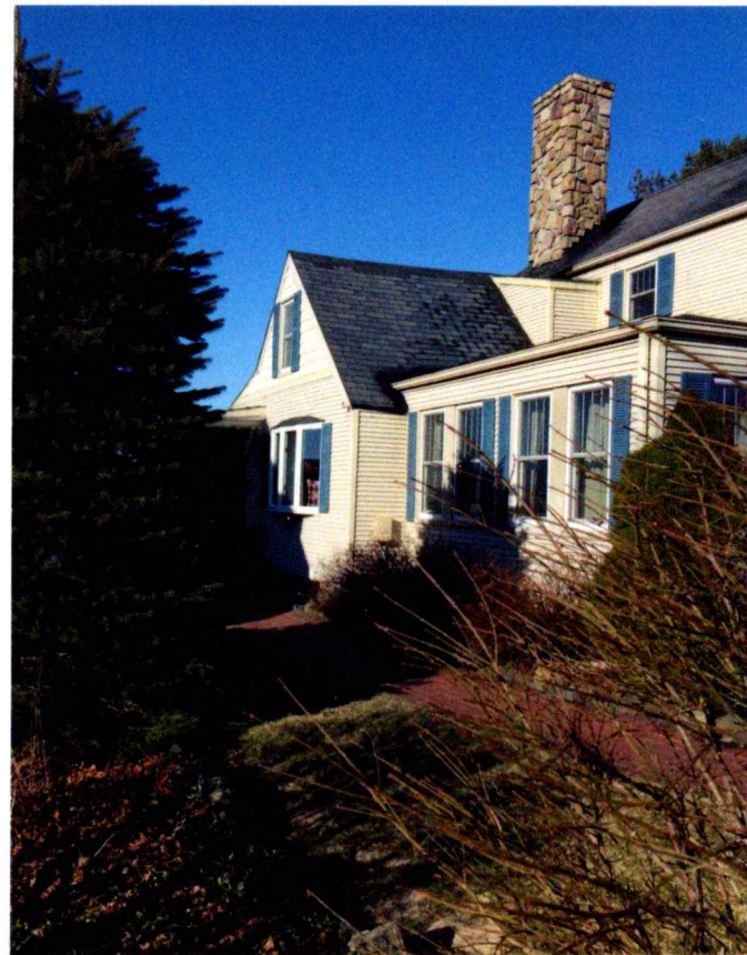
VIEW FROM LEFT SIDE YARD
