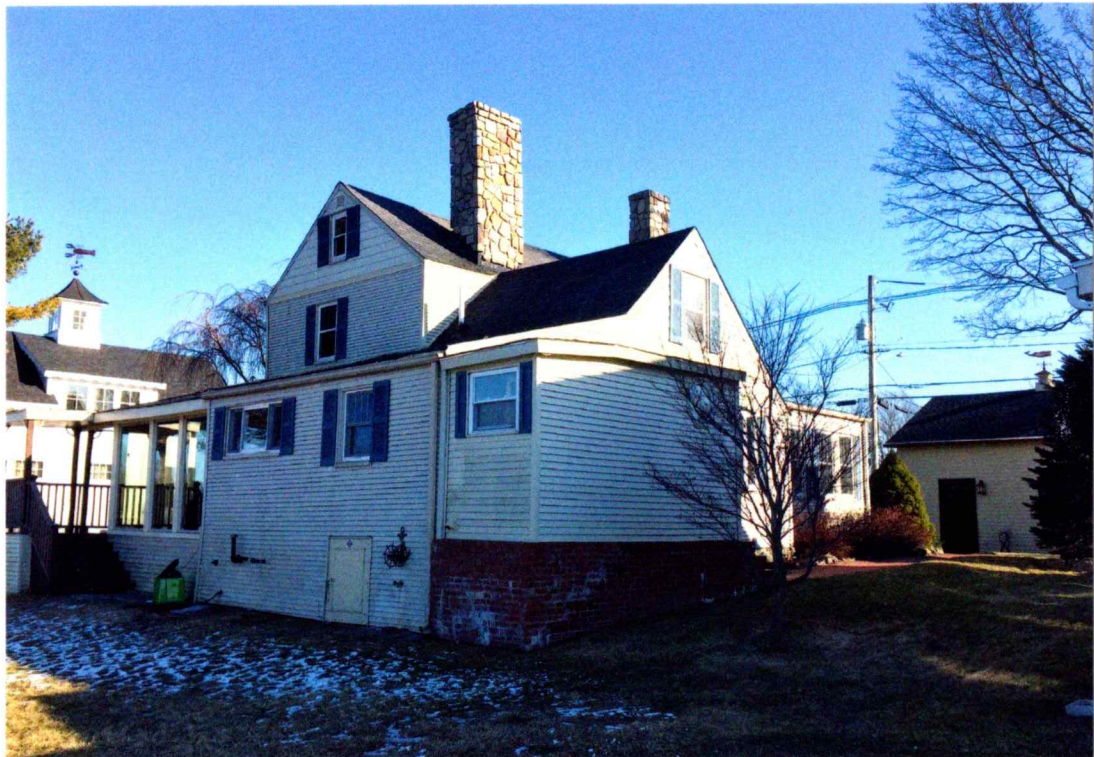
REAR VIEW FROM WEST
