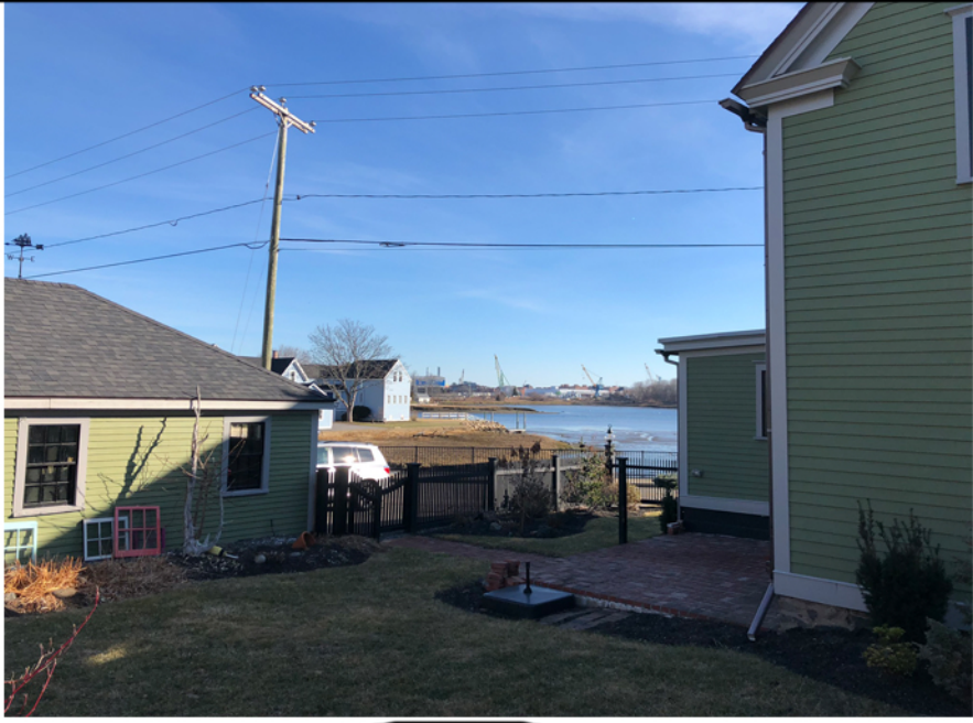
VIEW FROM BACK YARD
