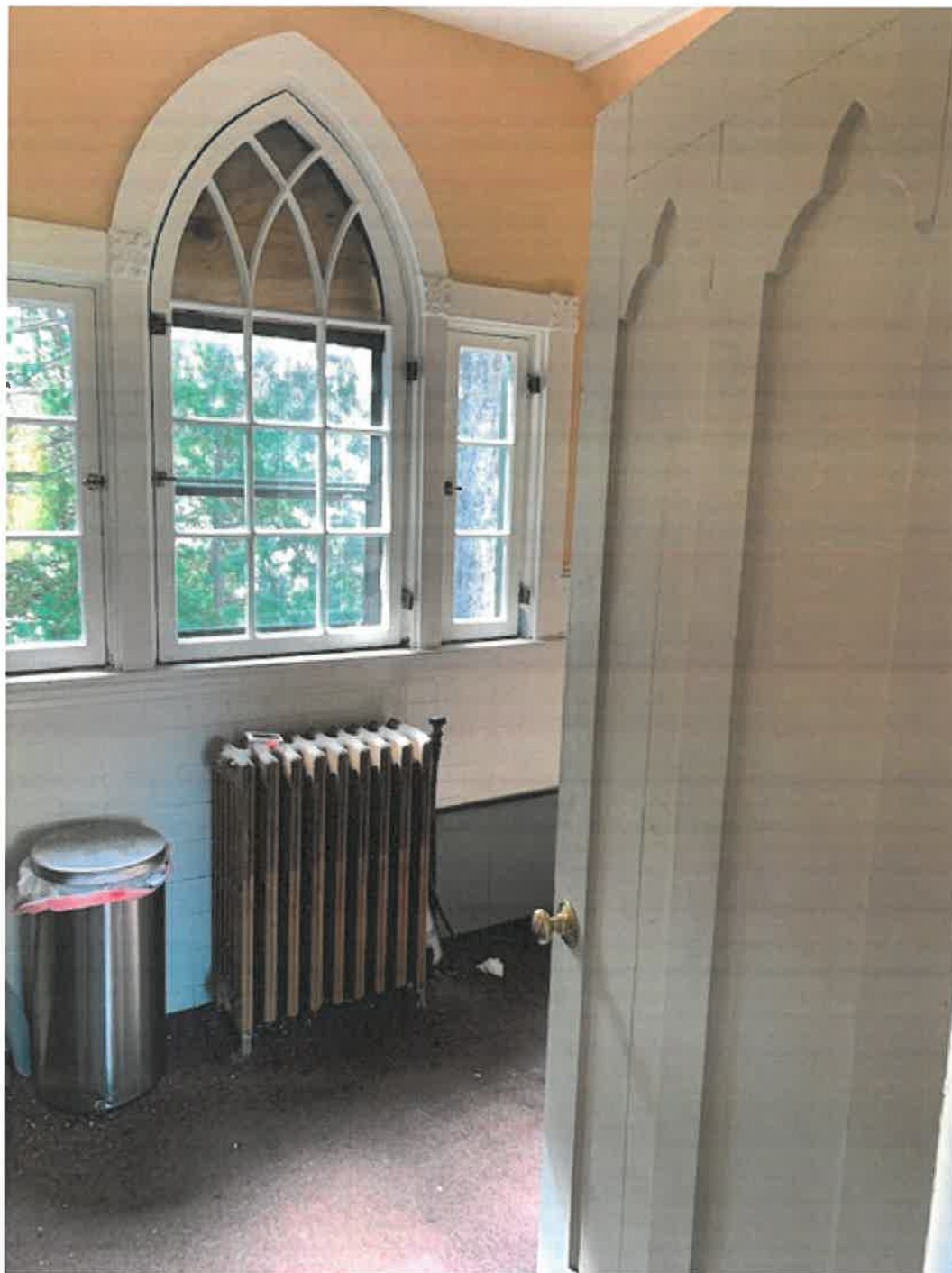
Existing second floor bath
