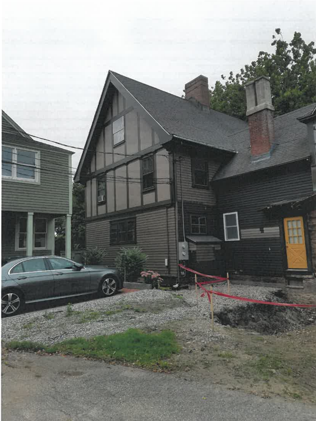
North side (Tudor structure) view from side yard
