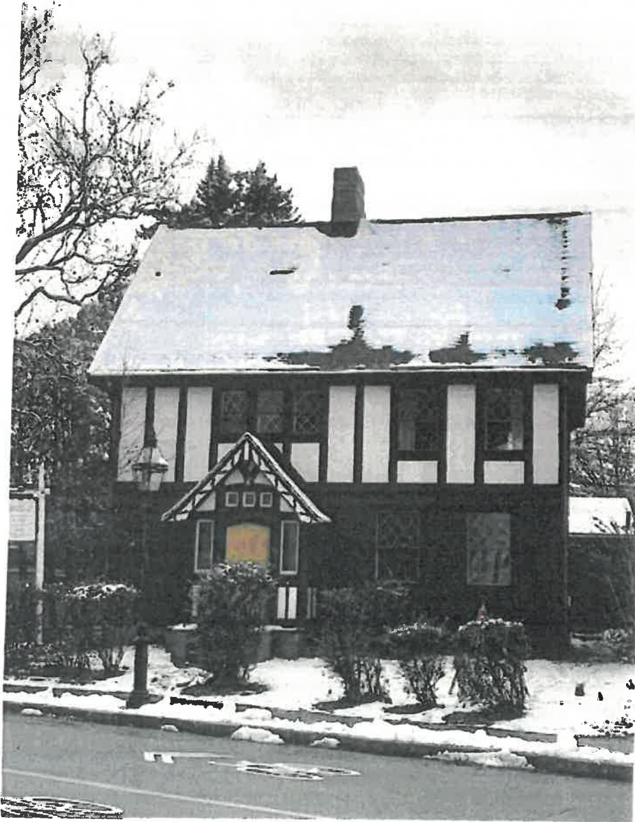
Front facade from Middle Street
