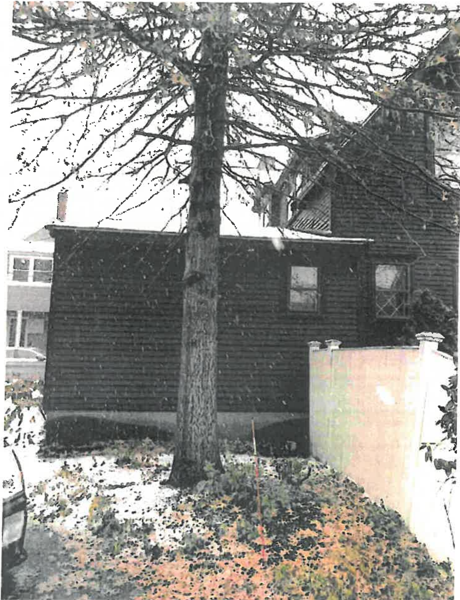
Rearview including addition to be removed and replaced
