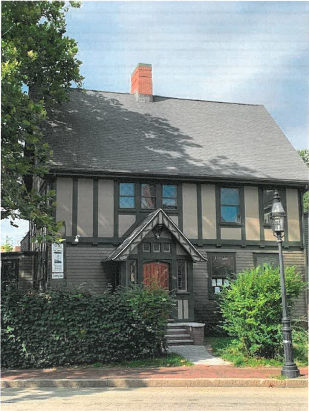
Front (East) façade from Middle Street
