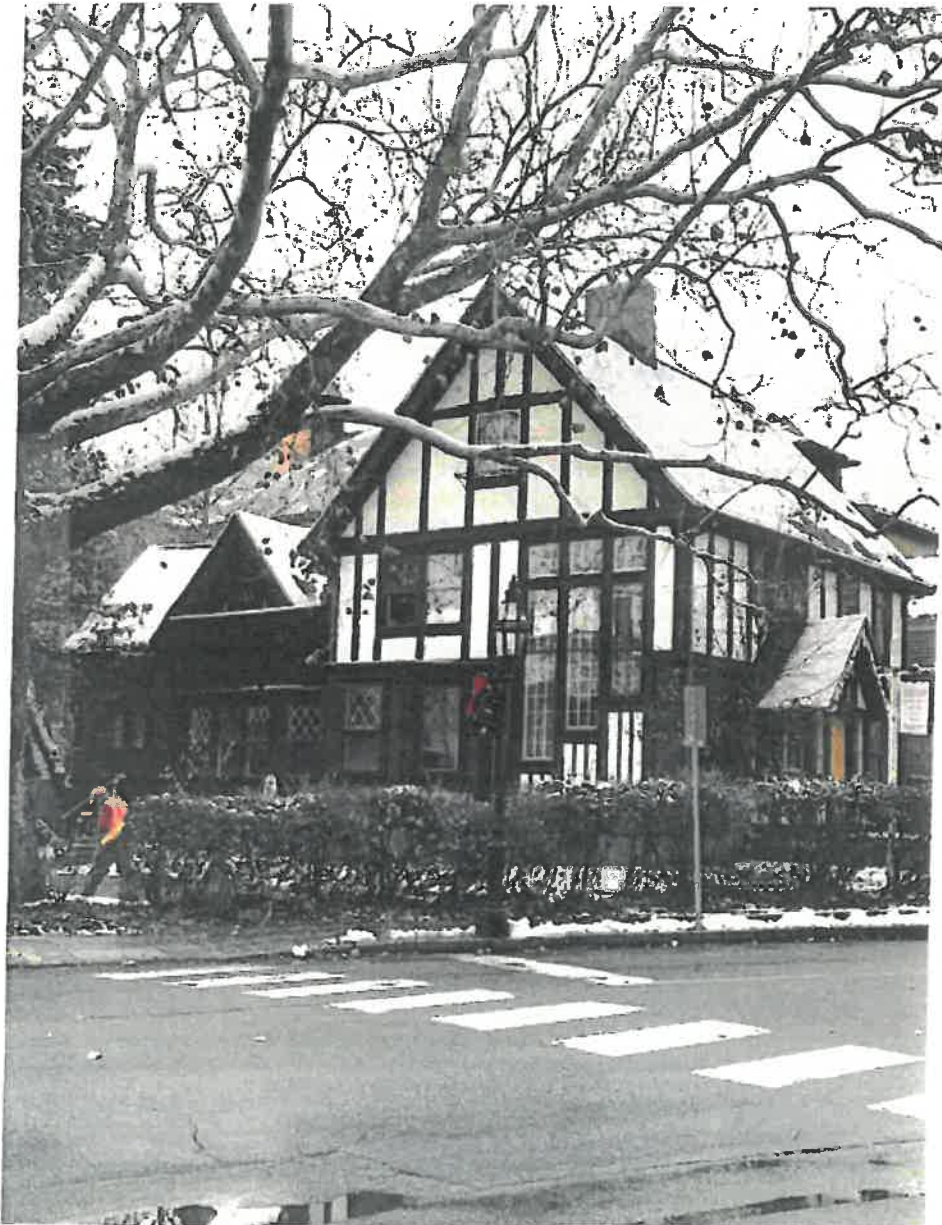
Front and left side view from State and Middle Streets intersection
