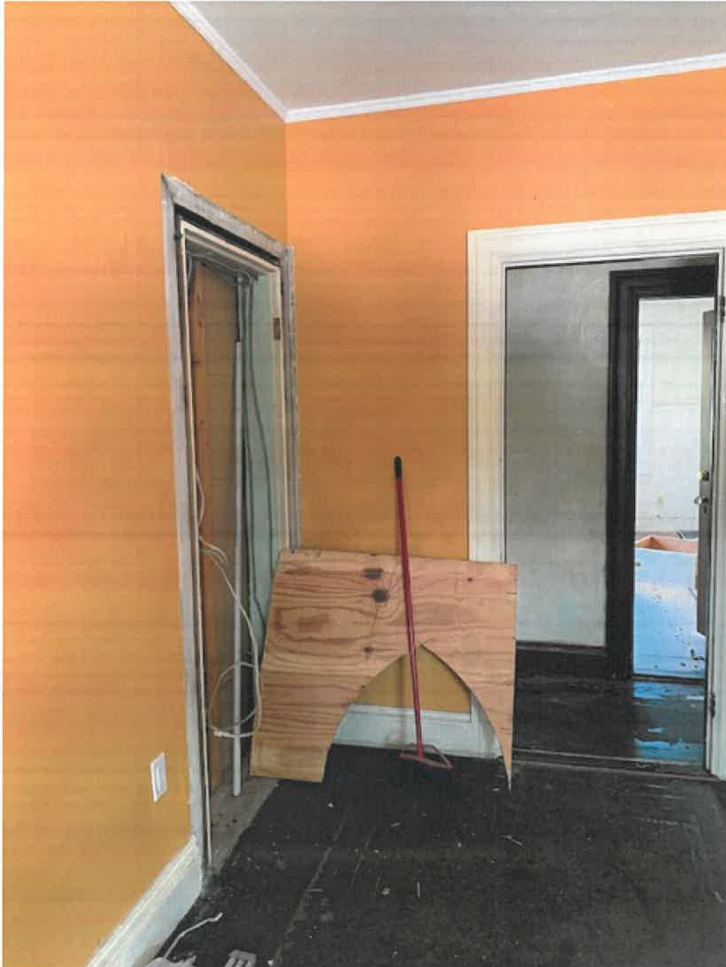
Another view of proposed second floor bedroom
