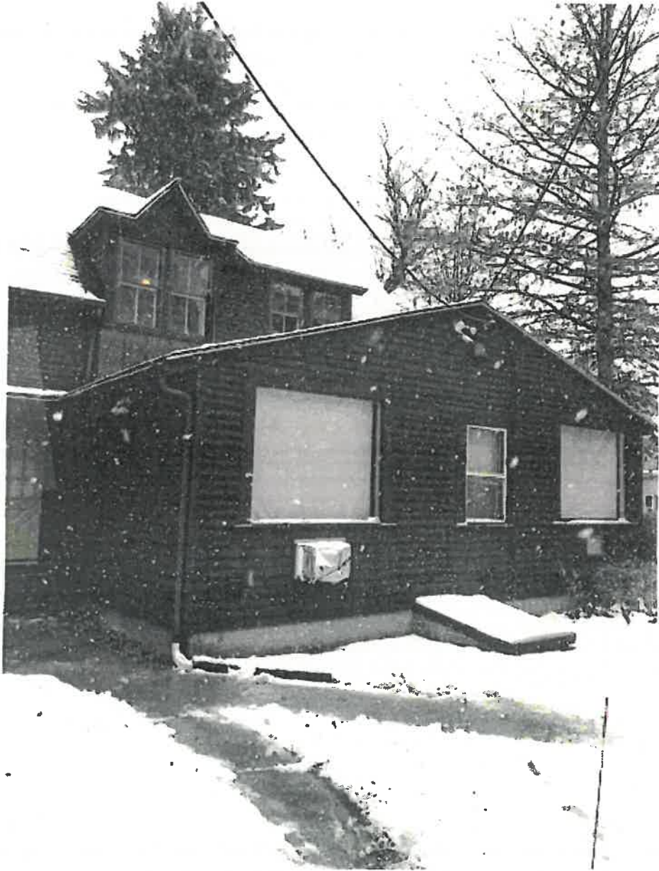
Right side view, including addition to be removed and replaced
