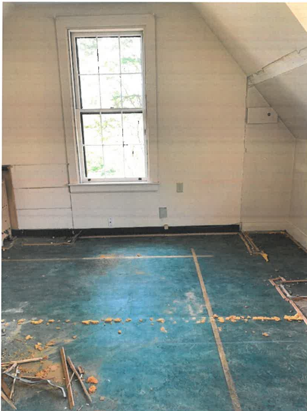
Second floor rear room
