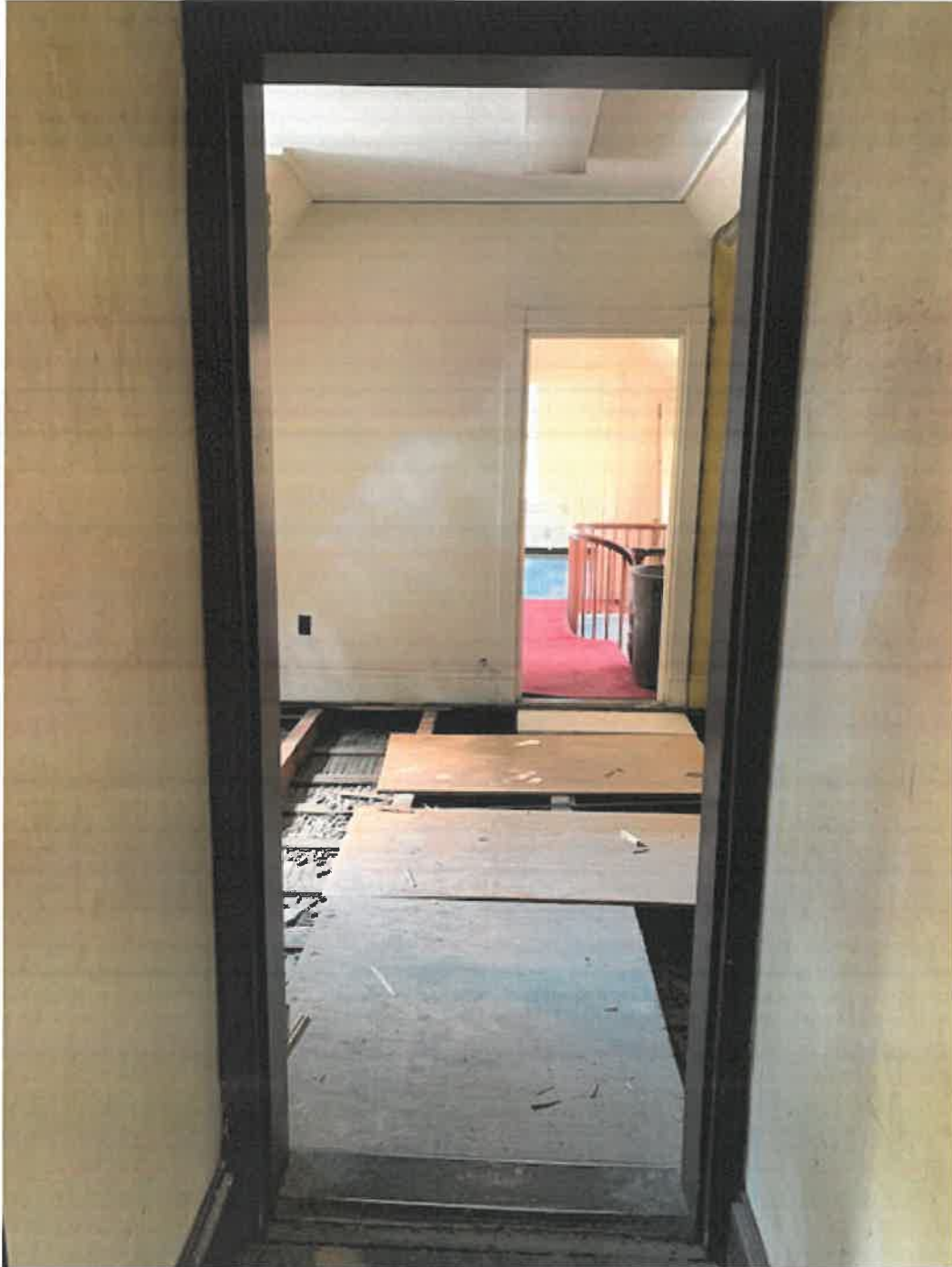
Second floor bath & laundry looking toward spiral staircase
