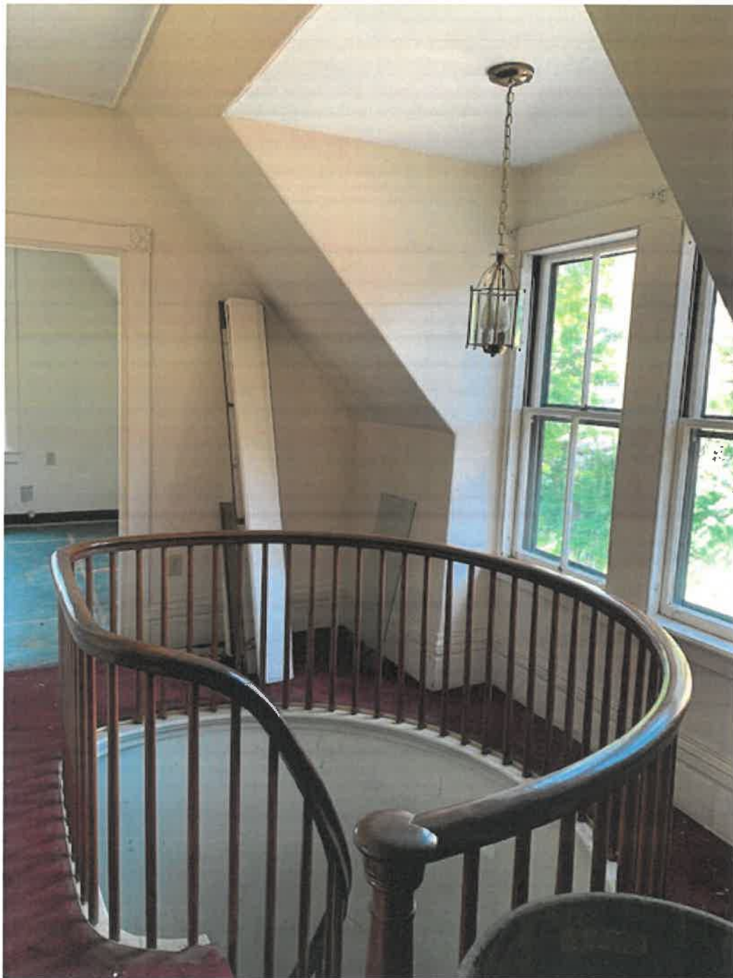
Second floor at top of spiral staircase
