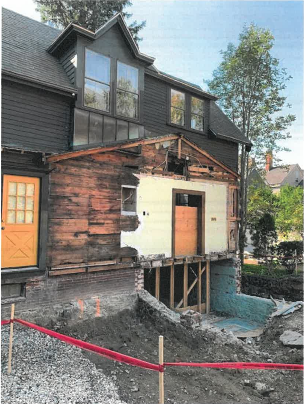
North side (Gothic structure without addition) view from side yard
