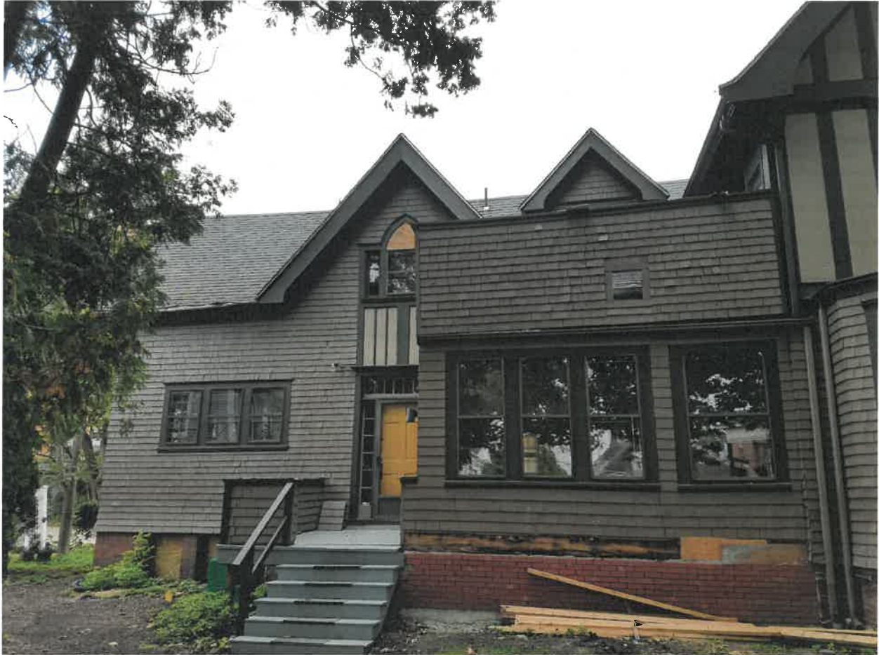
South side (Gothic addition) view from State Street
