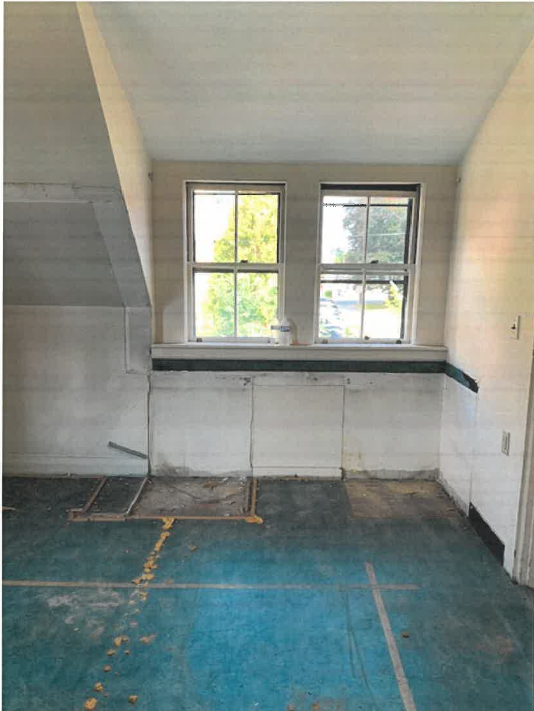
Second floor rear room
