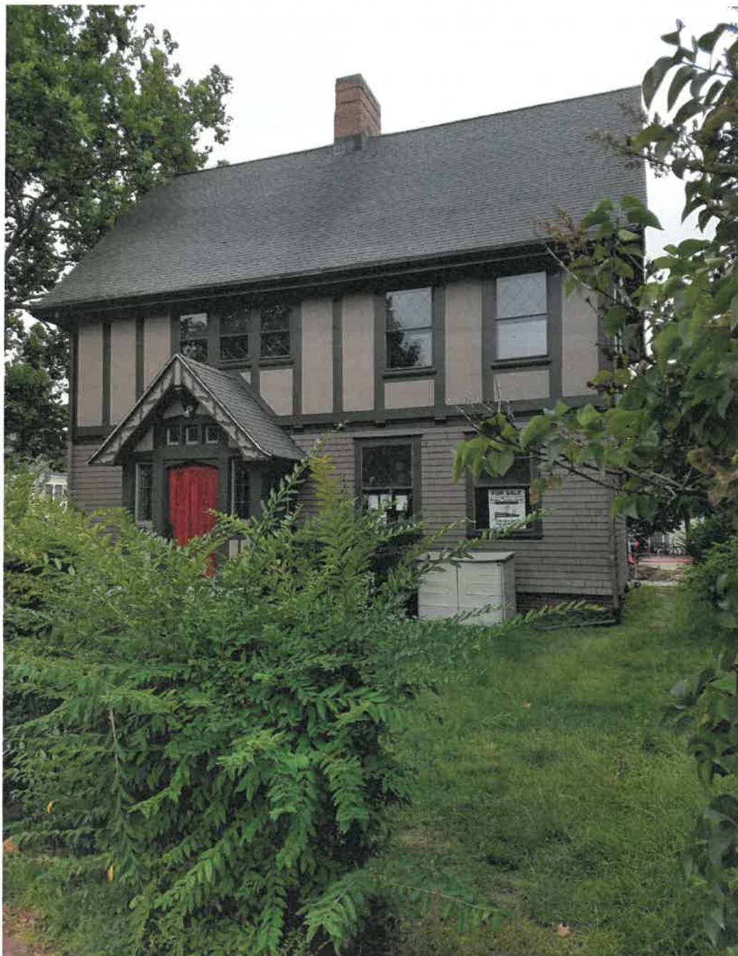
Front (East) façade from Middle Street
