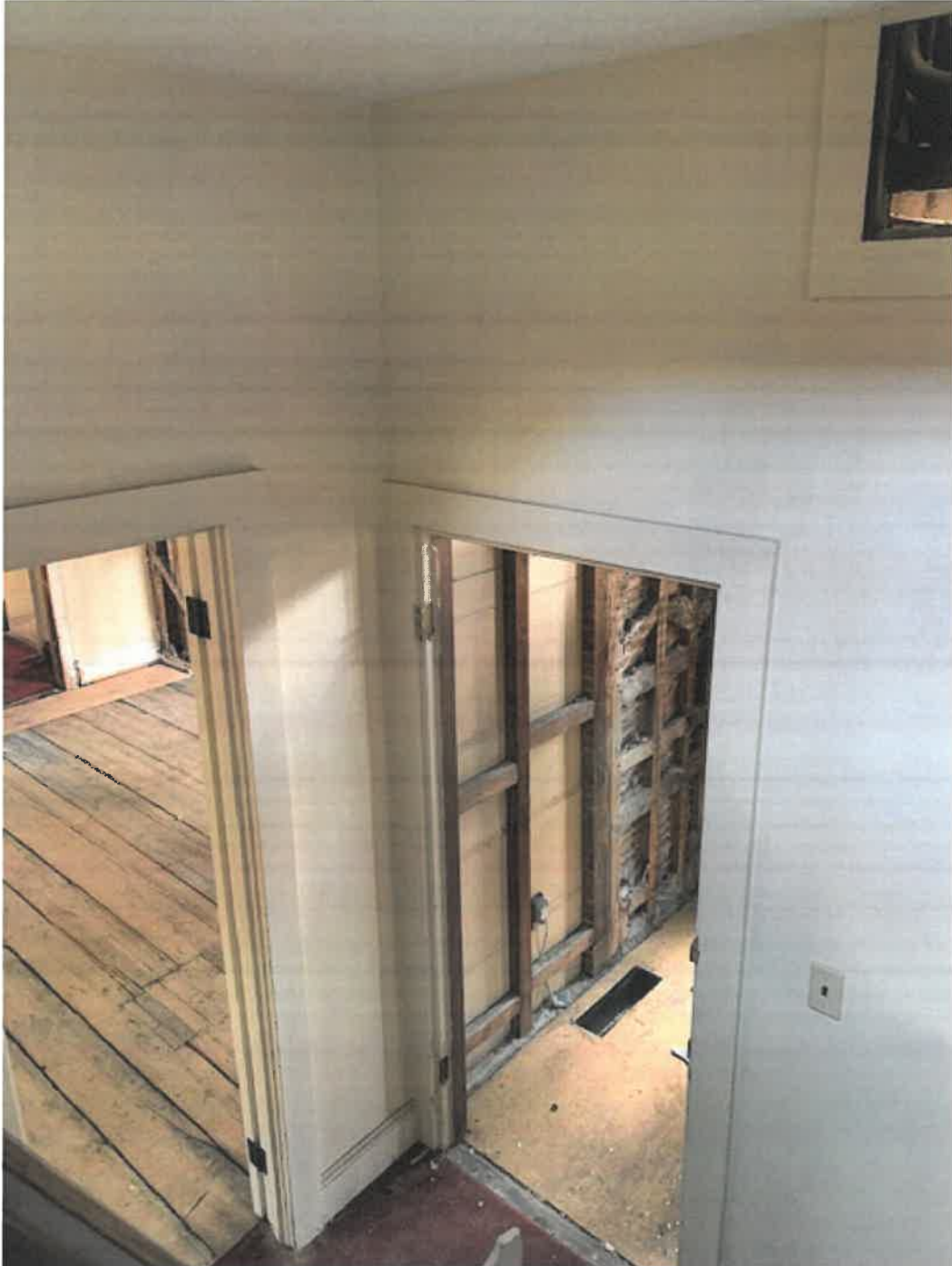
Second floor looking down spiral staircase
