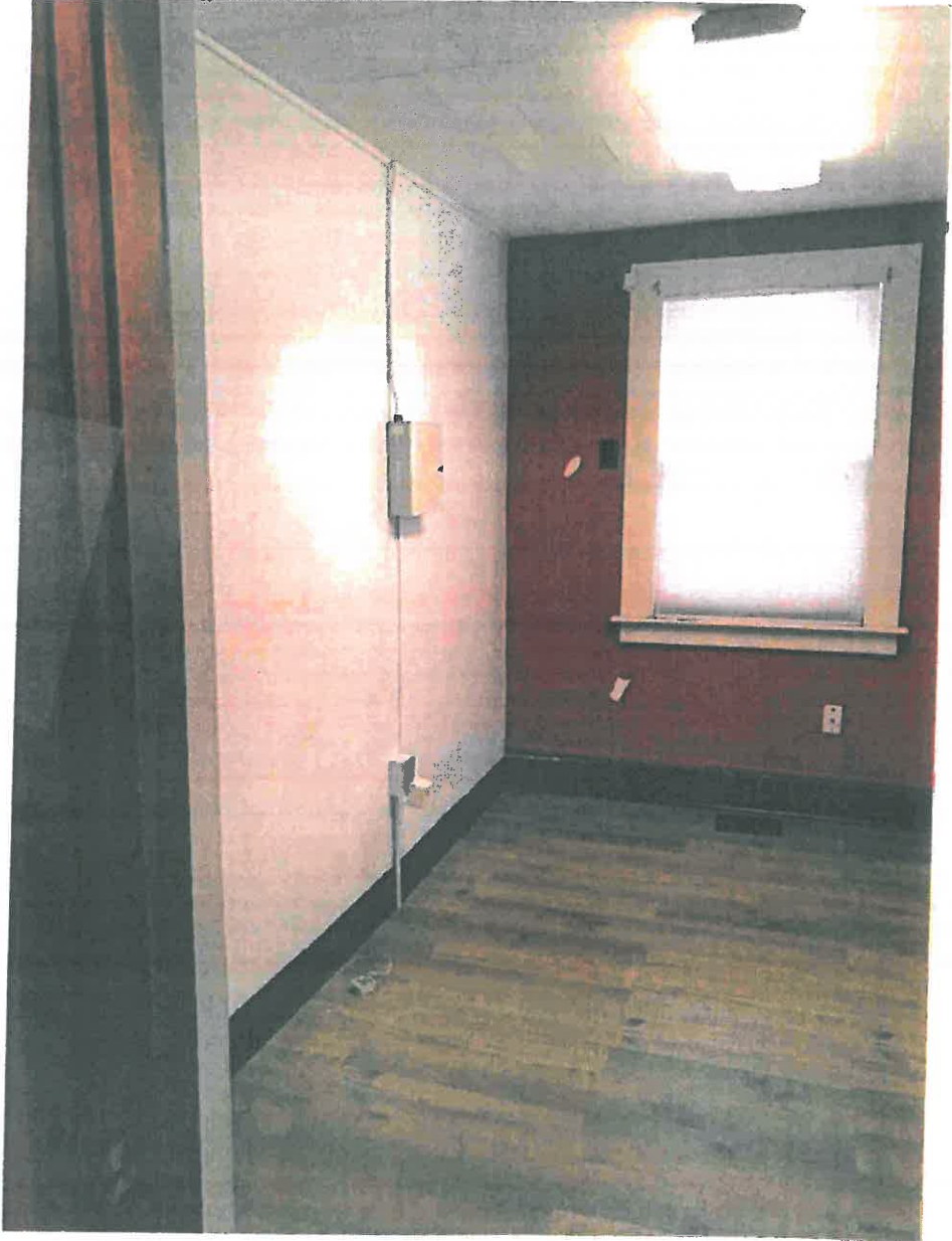
Interior – one-story rear addition
