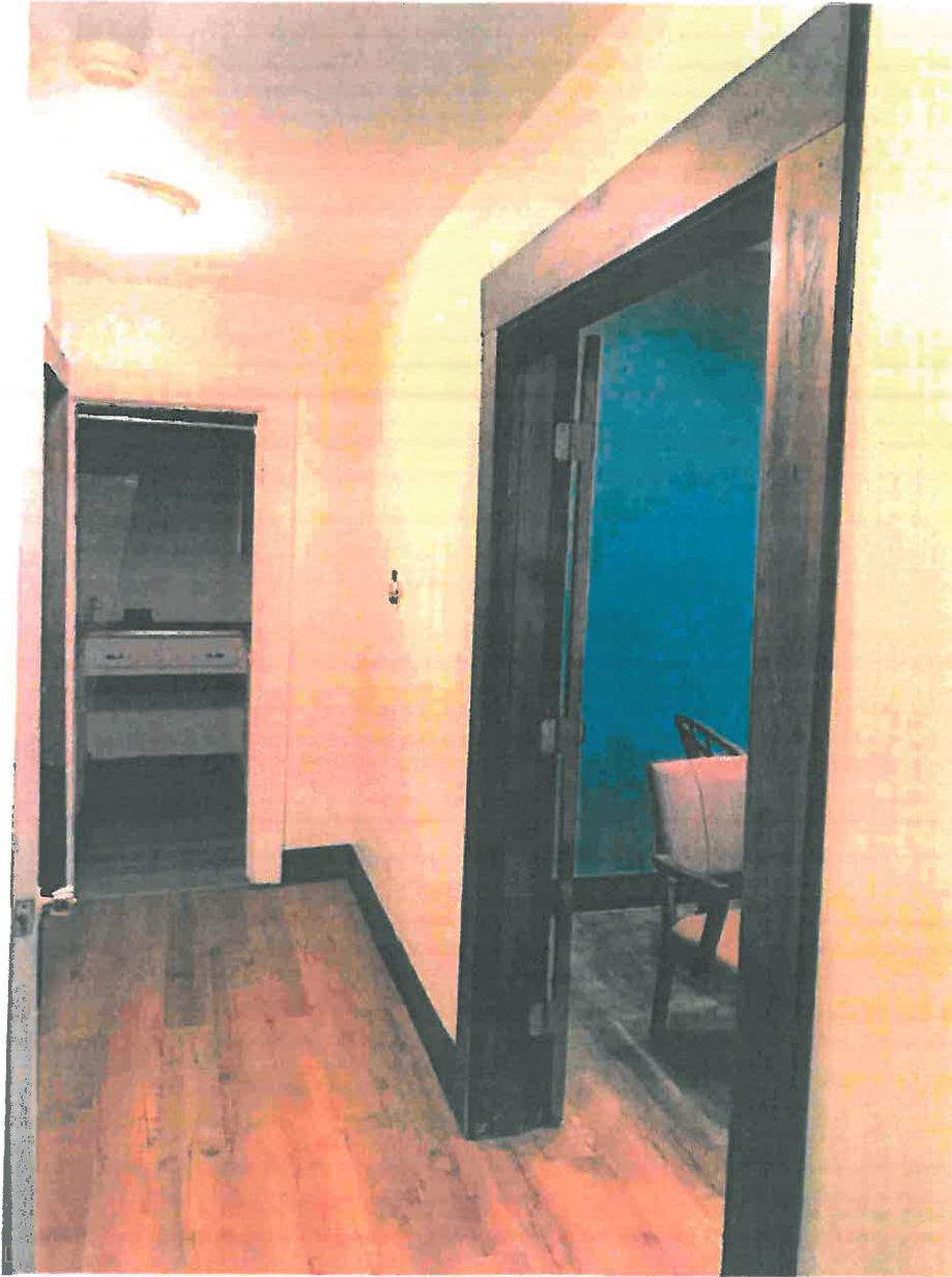
Interior – one-story rear addition
