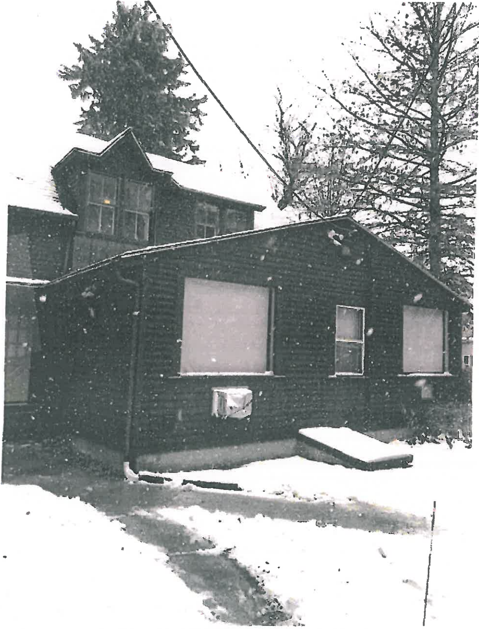
Right side view, including addition to be removed and replaced
