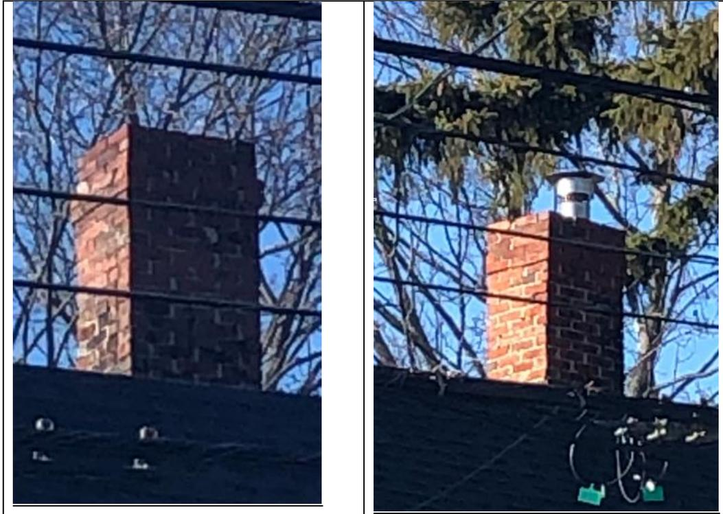
The chimneys currently lack support as the mortar is not holding them together, above the roof line. The right chimney is being used to vent the steam boiler and the hot water heater. The left chimney is being used to vent the hot water only.
