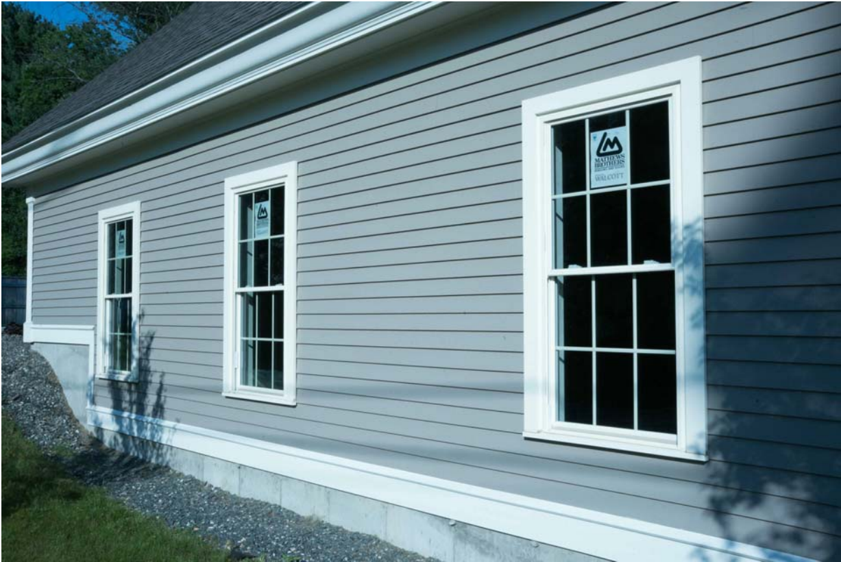
MATHEWS BROTHERS SPENCER WALCOTT PVC WINDOWS TO REPLACE ALL EXISTING VINYL WINDOWS (DOUBLE HUNG SHOWN) - REFER TO APPENDIX 01
