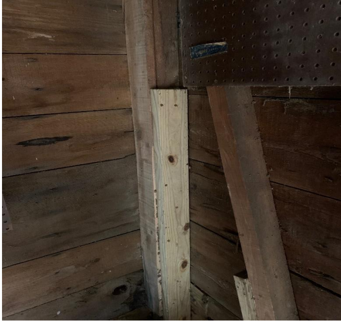
Temporary supports to stabilize corner posts
