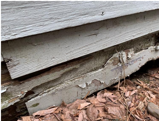
Collapse of subfloor visible from exterior rear of shed
