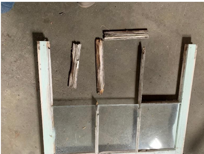
Lower window sash removed to show degree of wood rot
