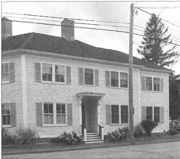
The massing and materials at this new building are similar to historic buildings in the area, however the design would be more sympathetic if the shutters were sized to fit the window openings and if the windows were separated.
