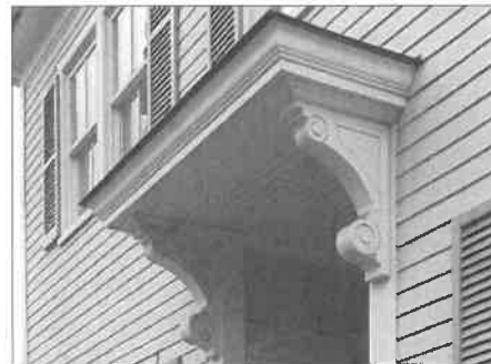
This wood bracketed door hood is located on a new building. The details represent a simplified interpretation of a Victorian-period door hood.
