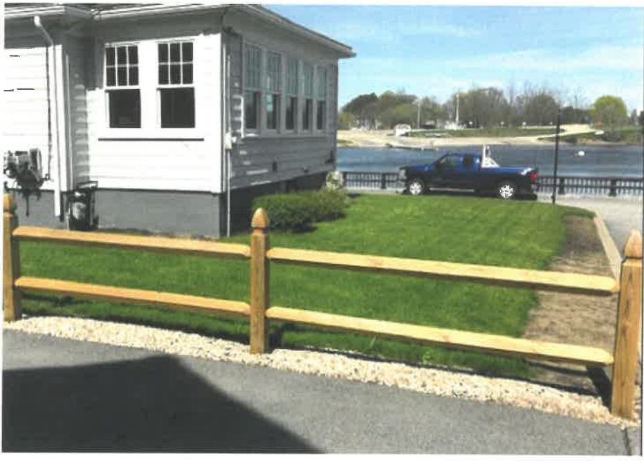
EXISTING 2-RAIL FENCE
