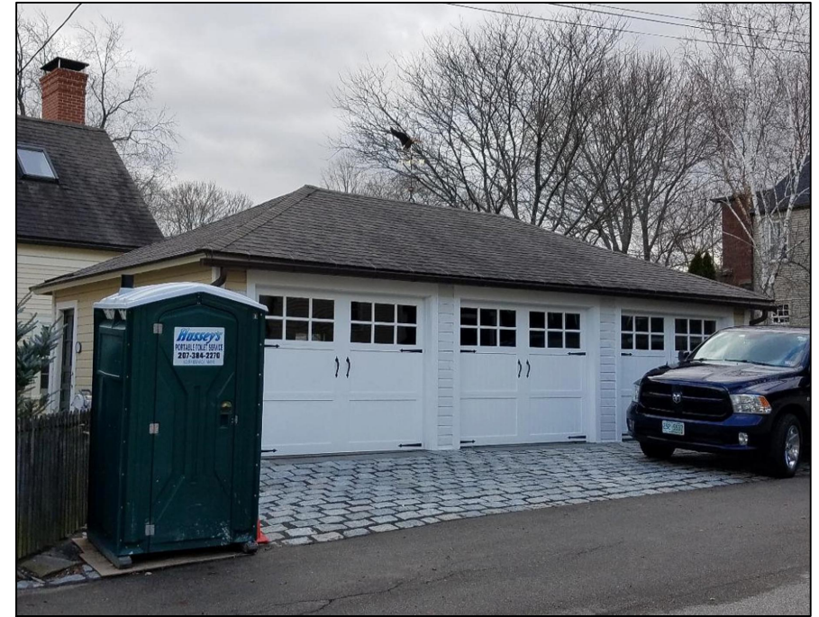
MARCY STREET GARAGE
