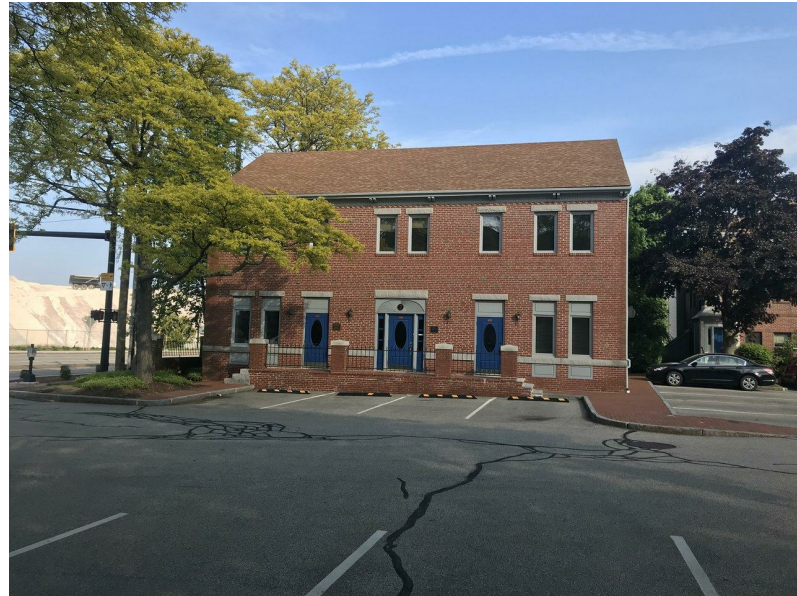
EXISTING/CURRENT SOUTH ELEVATION FROM ACROSS PARKING LOT
