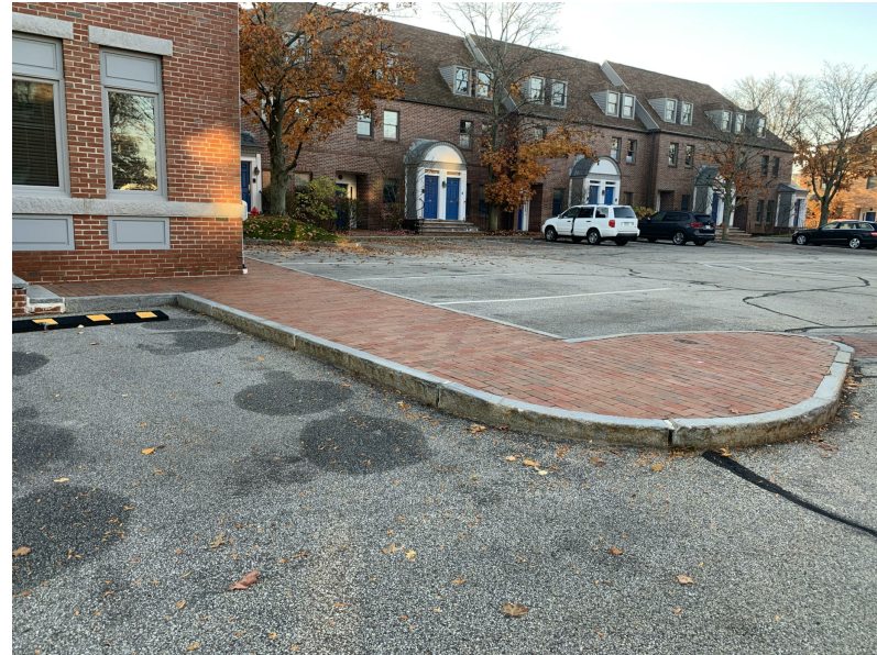
VIEW FROM WEST SIDE OF PROPOSED RAMP TO EAST SIDE OF EXISTING/CURRENT BUILDINGS IN COMPLEX
