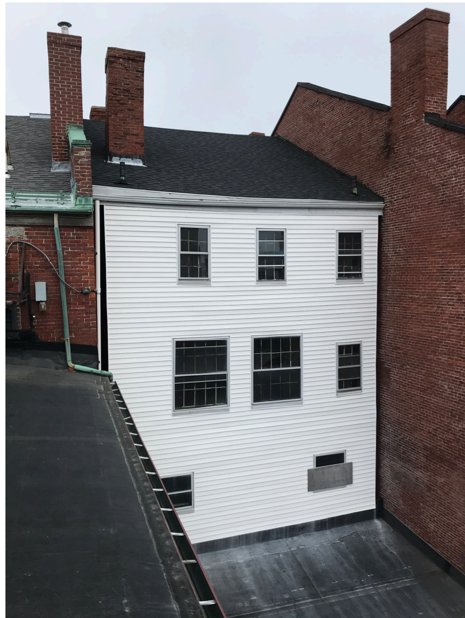
Existing East Elevation (Opposite Market St)
