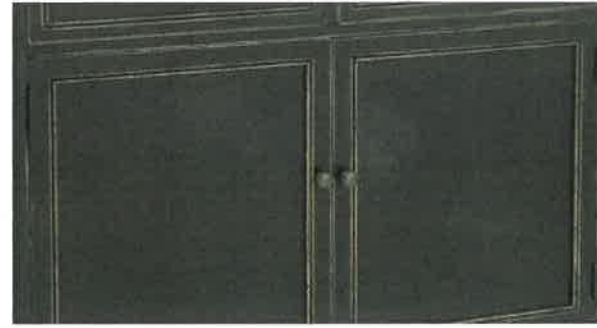
Bronze-colored exterior woodwork/ wood storefront with gold glaze
