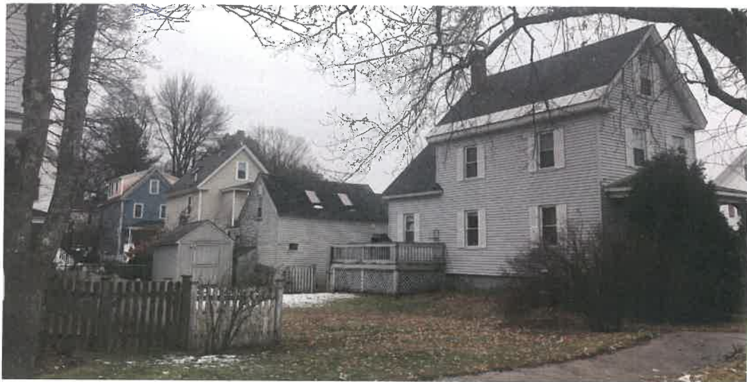
EXISTING CONDITIONS – VIEWED FROM NORTHEAST
