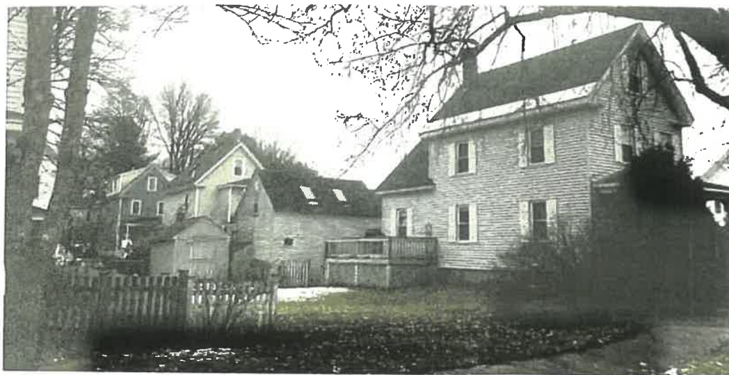
EXISTING CONDITIONS – VIEWED FROM NORTHEAST
