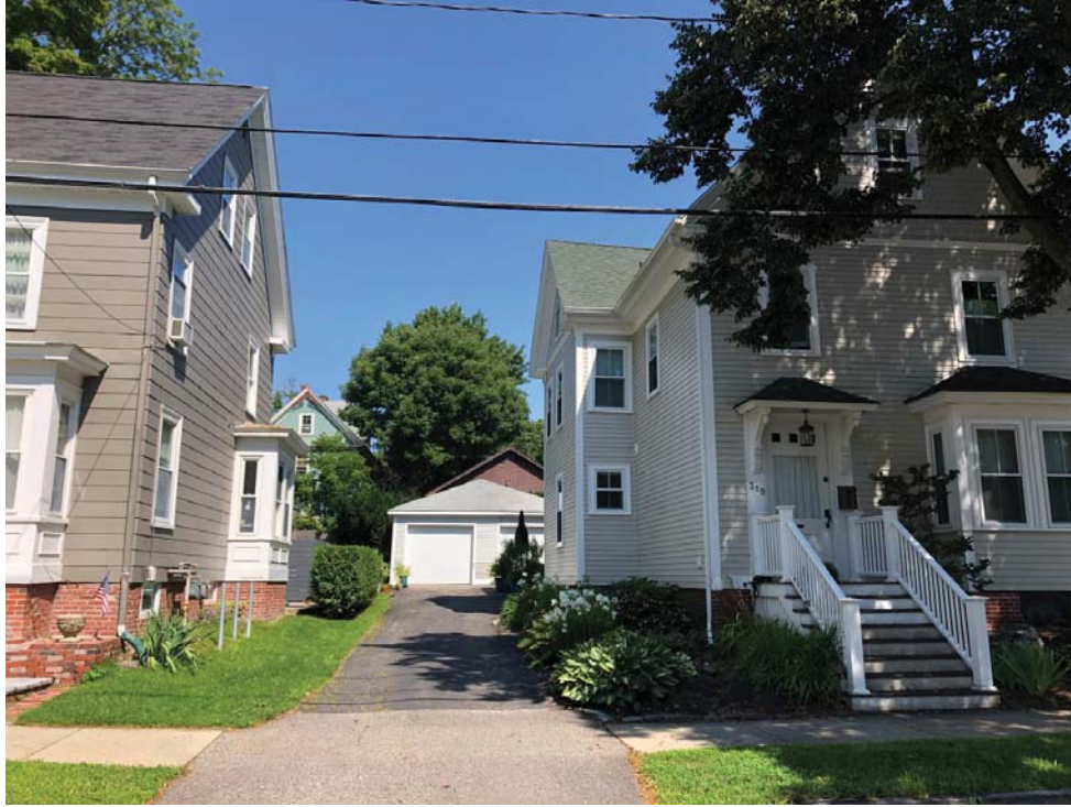
SOUTH ELEVATION FROM STREET
