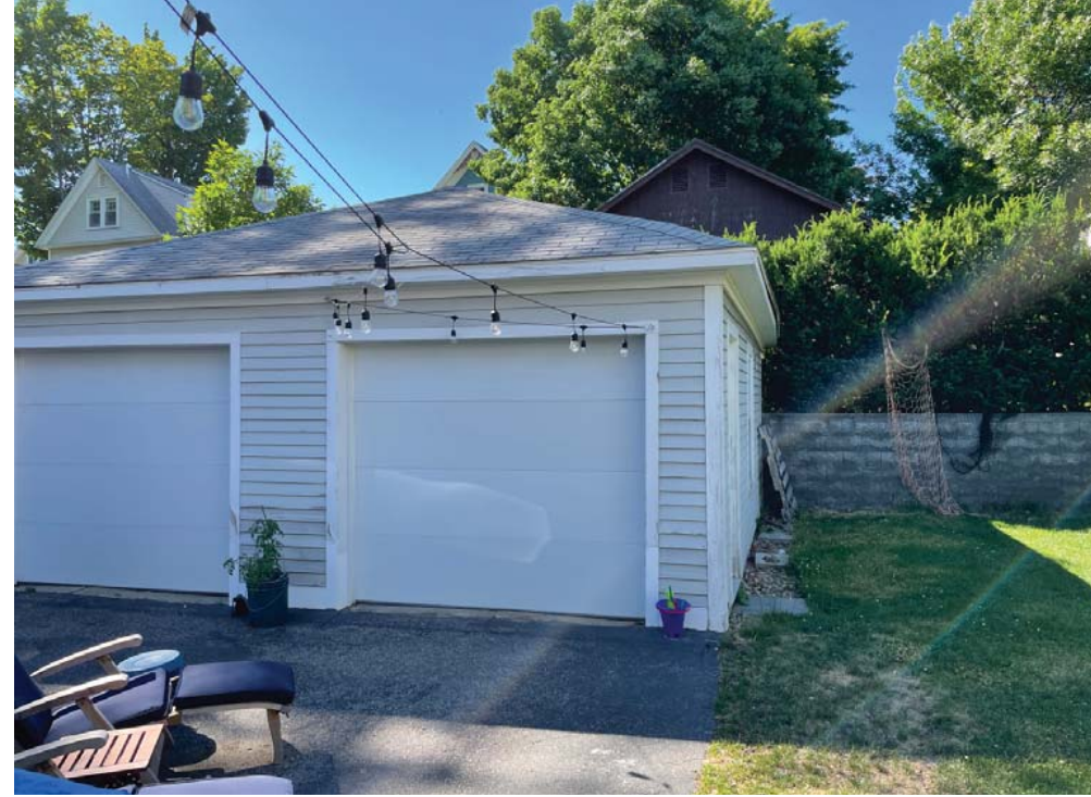
SOUTH EAST CORNER OF EXISTING GARAGE
