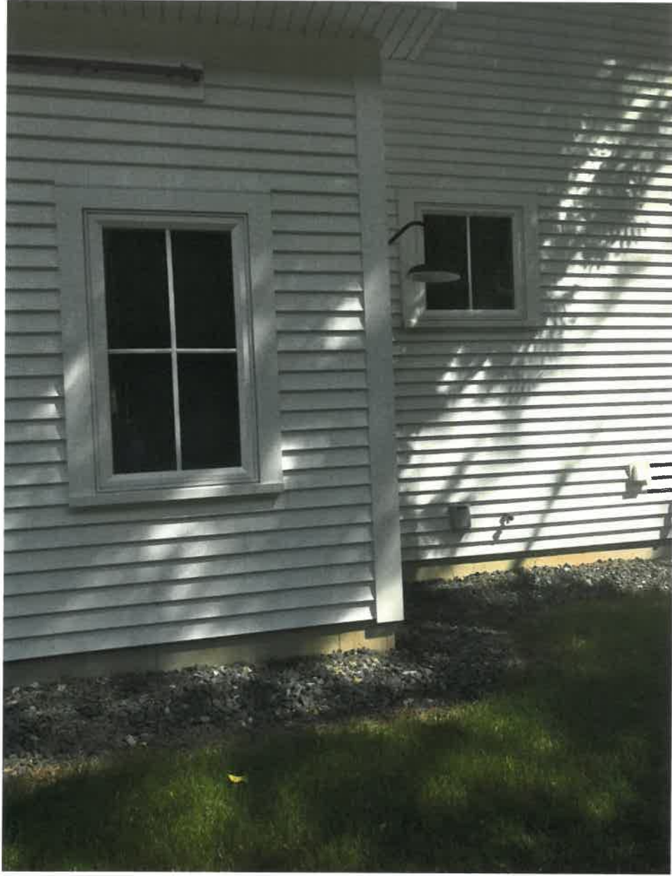
Casement at 4 Lydia; also shows soffit and corner board
