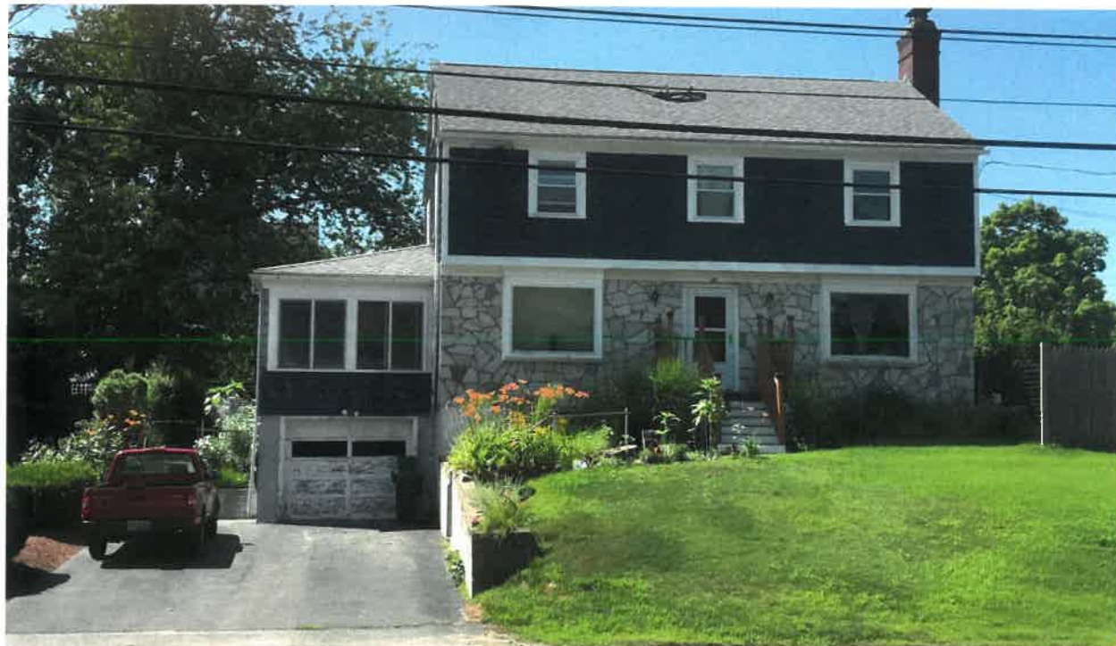
Context-Garrison across the street to the right
