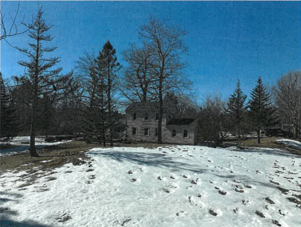
Existing Conditions – View of Property from the South
