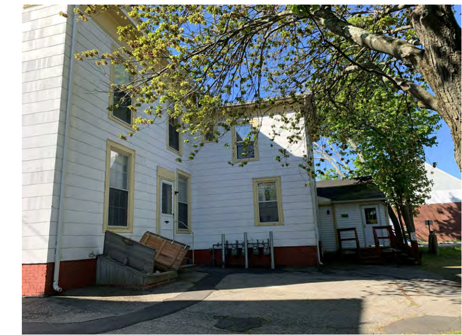
REAR (FROM NORTHEAST)
