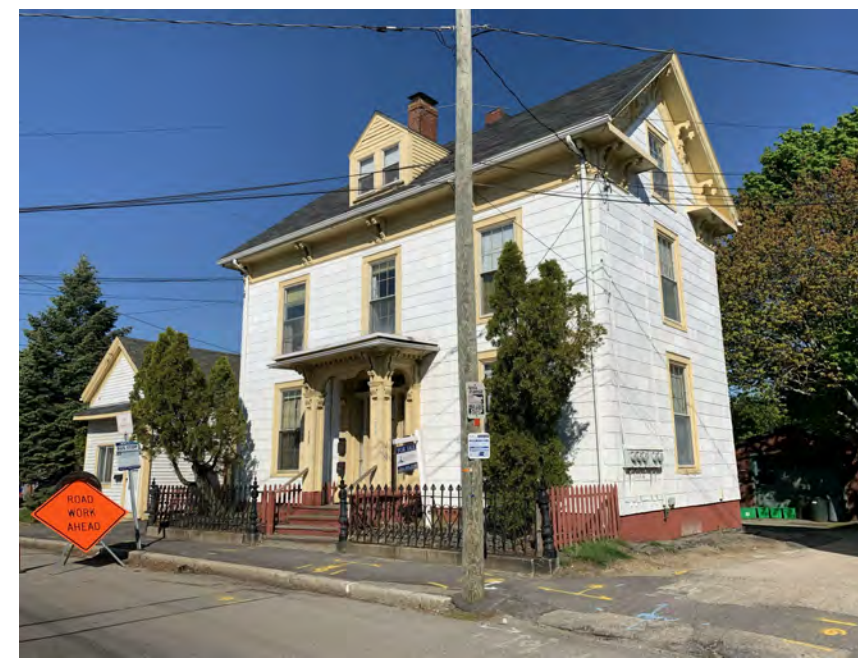
FRONT (FROM SOUTHEAST)
