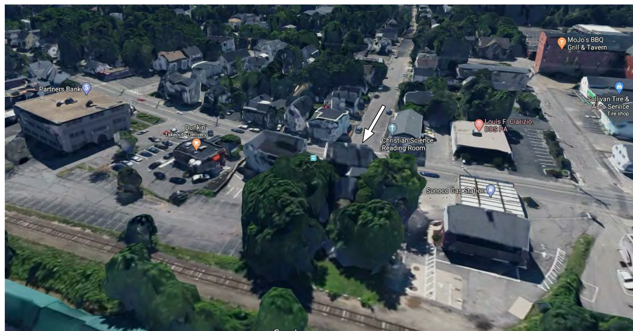
AERIAL BIRDSEYE VIEW (FROM SOUTHEAST)
