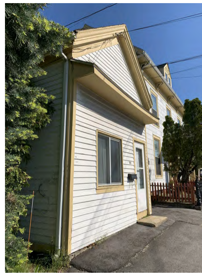
UNIT 559-1 - FRONT (FROM SOUTHWEST)
