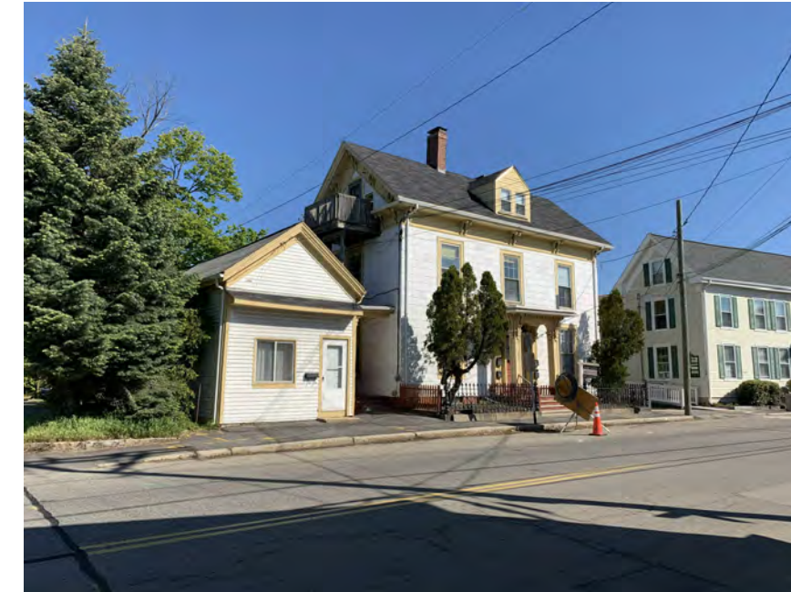
FRONT (FROM SOUTHWEST)
