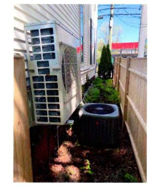
Lower Exist Heat Pump & Add single Heat Pump, relocated from Right Side. The 2 Exist Units on the Right Side will be replaced with 1 Unit. Both will be ground mounted. Exist AC Condensor to remain.
