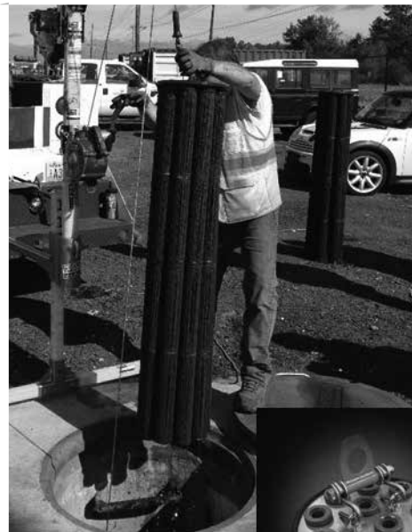
Cartridge Removal & Lifting Device
