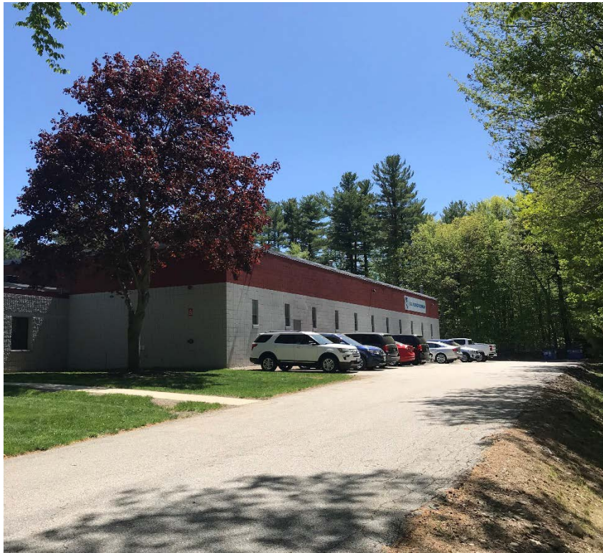
View from Property from the side (north)
