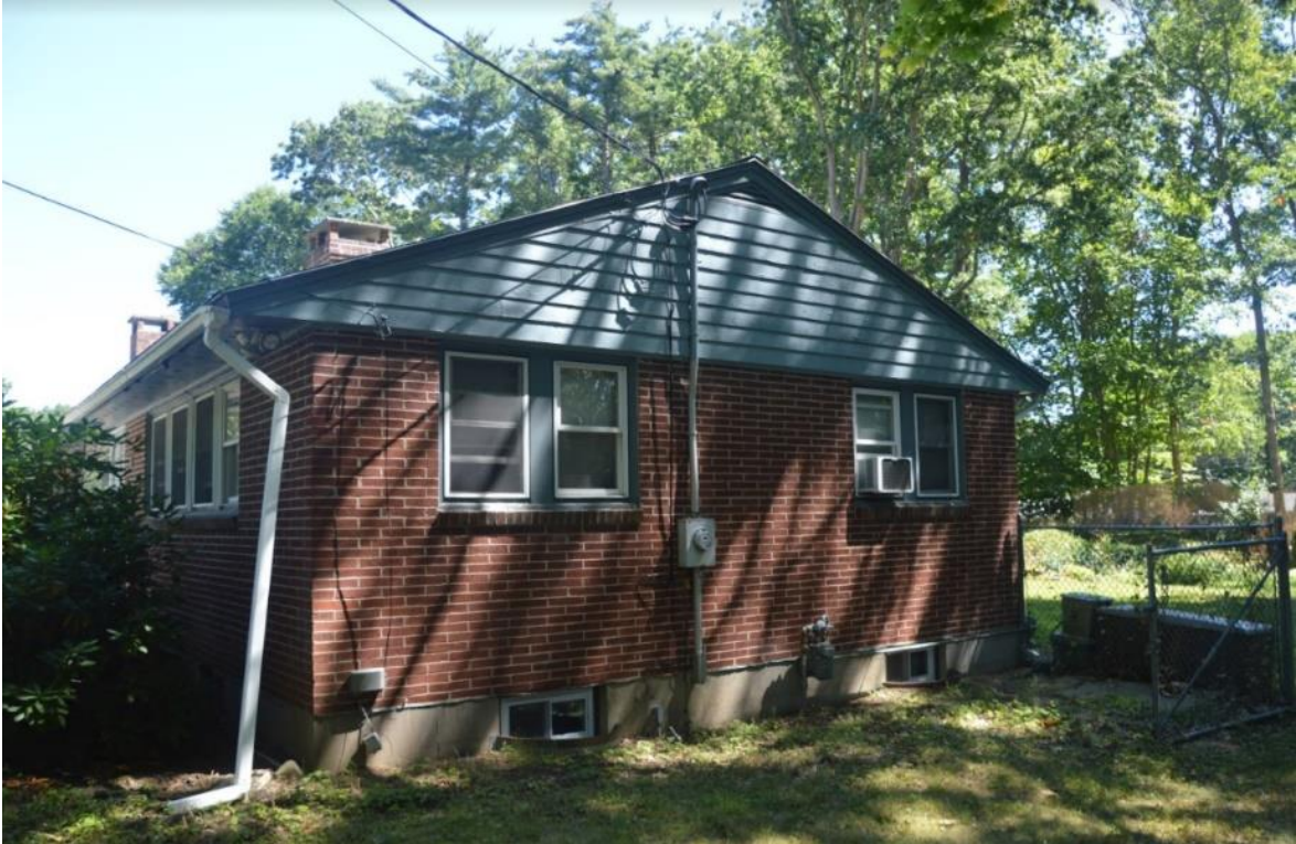
Right side of existing home from Grant Ave (southern side)
