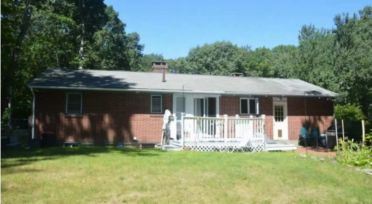
Back Side of existing home (East side)
