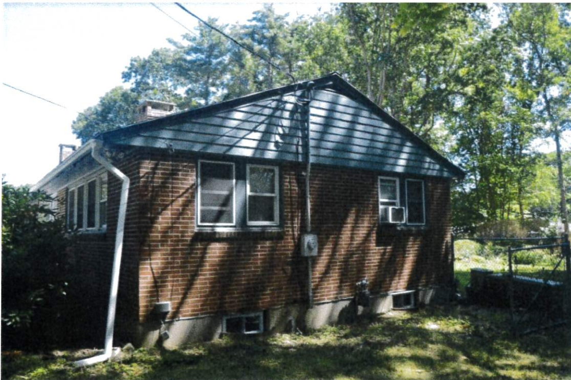
Right side of existing home from Grant Ave (southern side)
