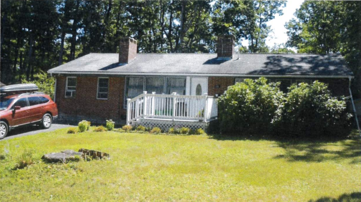
Front of existing home from Grant Ave
