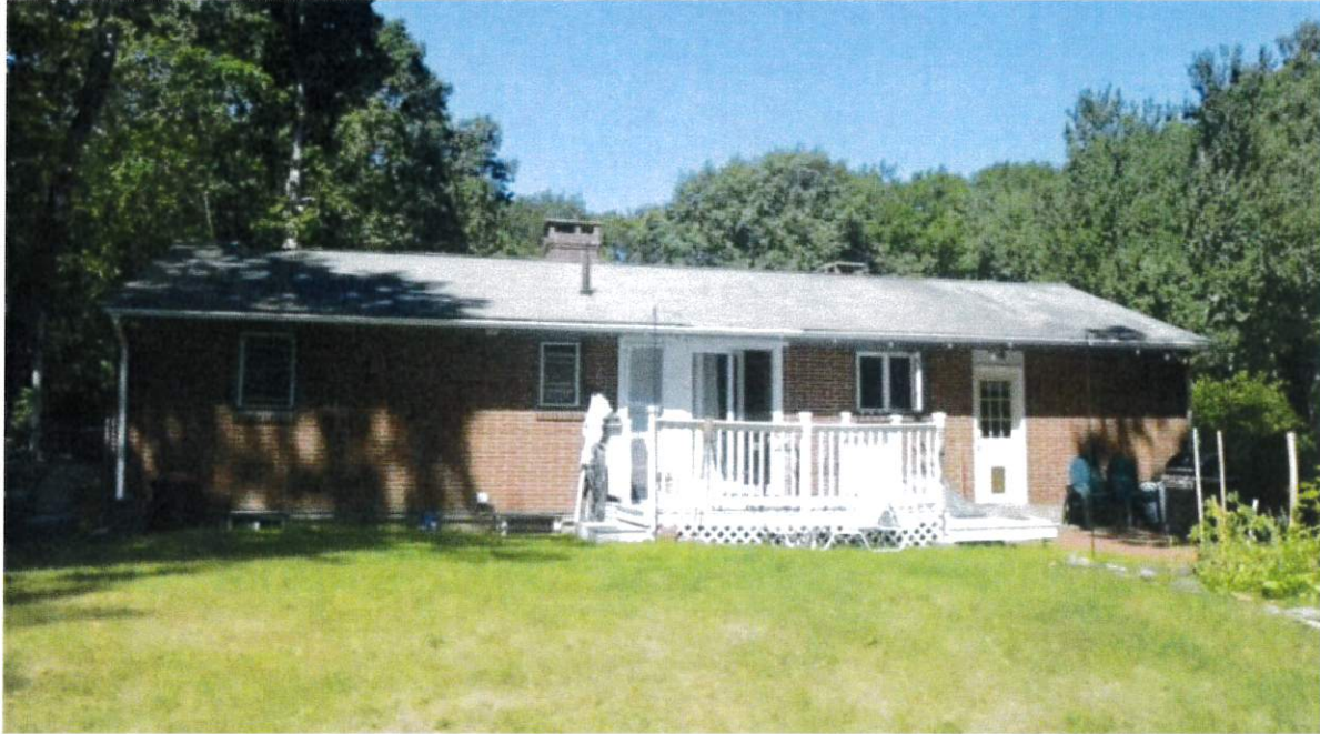
Back Side of existing home (East side)
