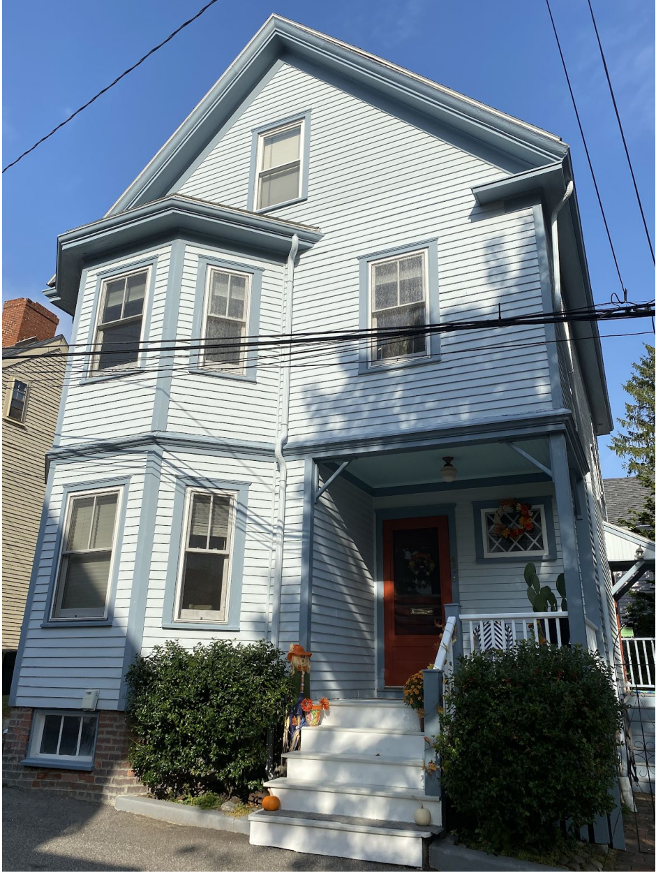
No changes to front facing Gardner St.
