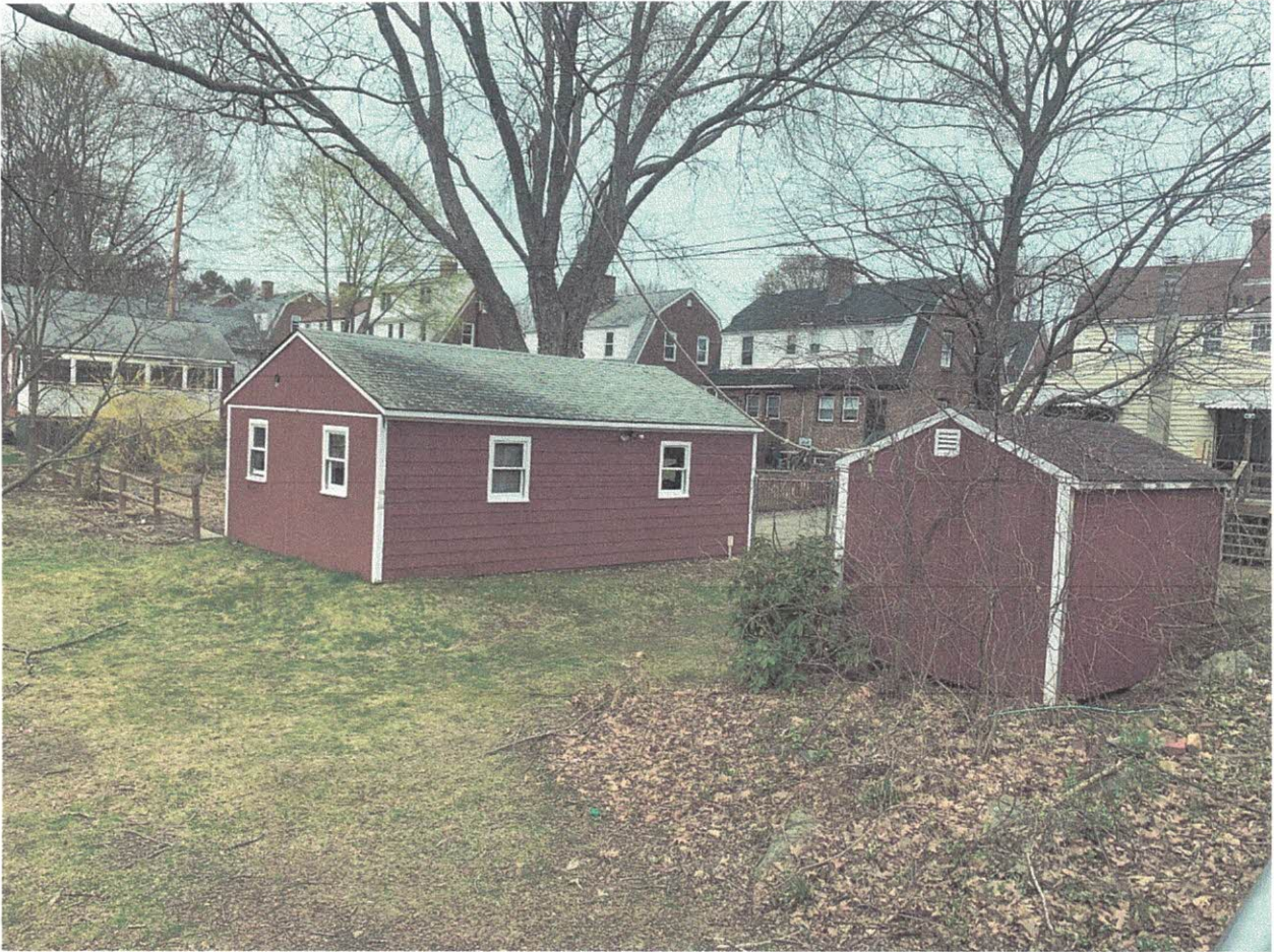
Alternate View of Garage and Shed
