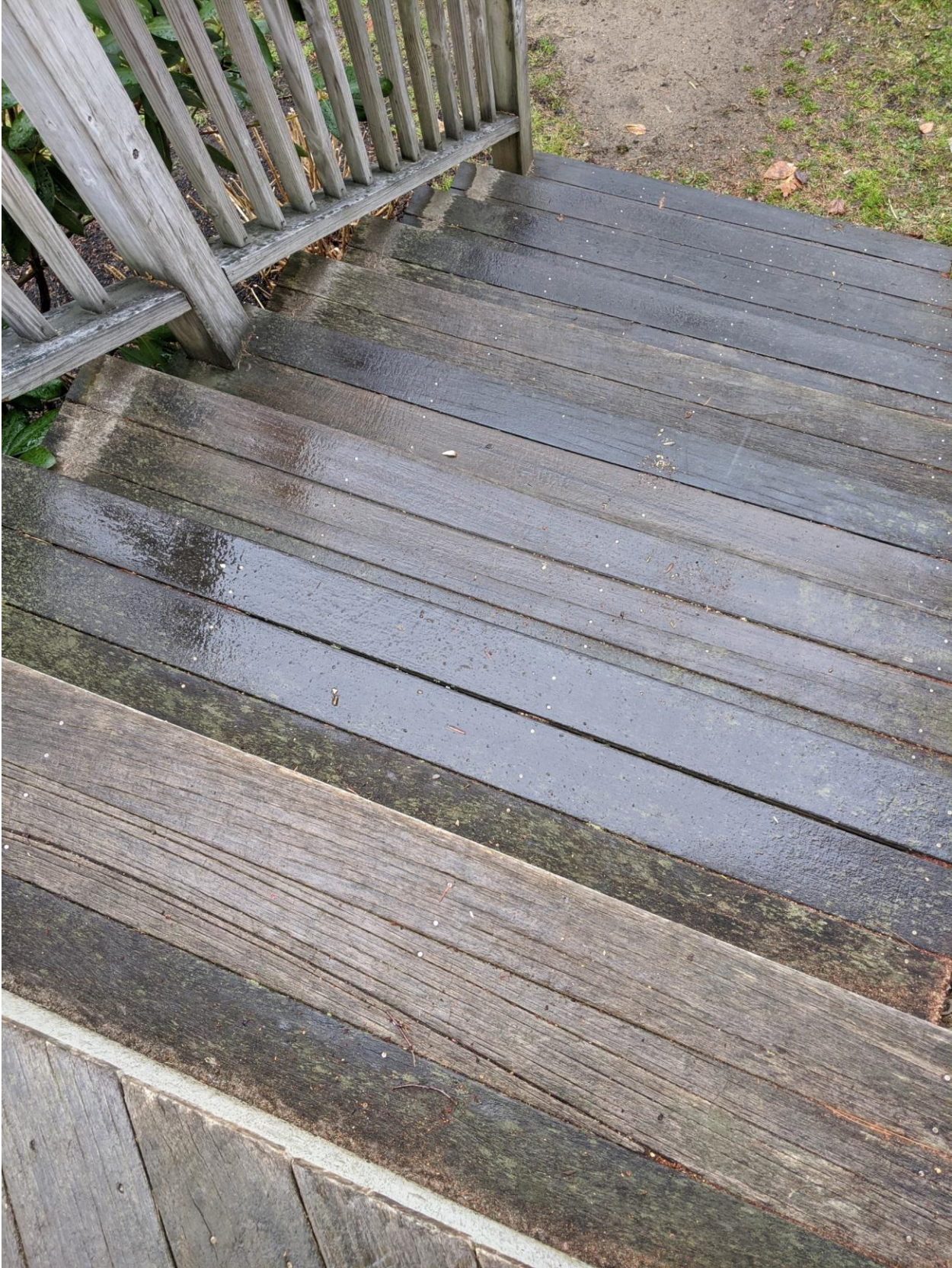
Existing Deck – Photo 3
