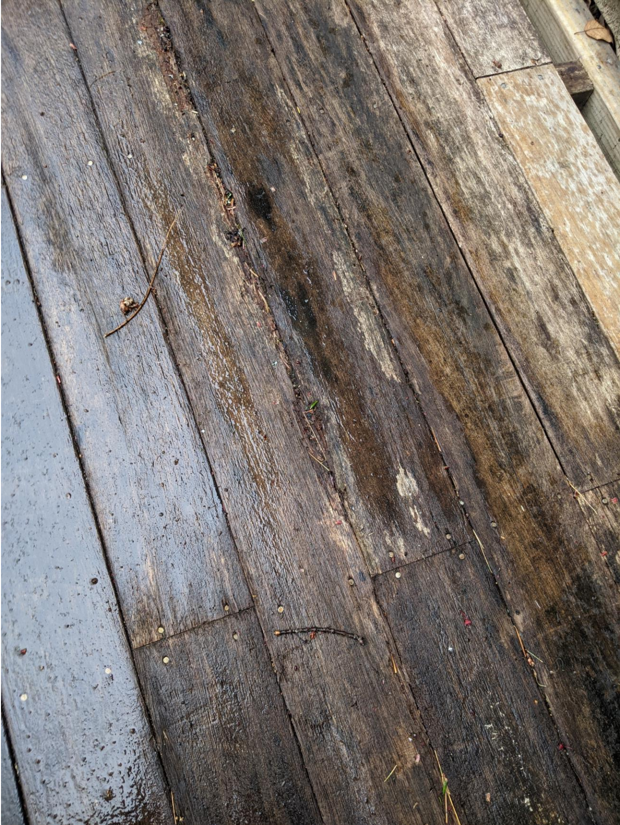
Existing Deck – Photo 1
