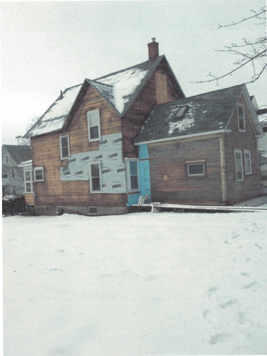
Southerly Side of Existing House
