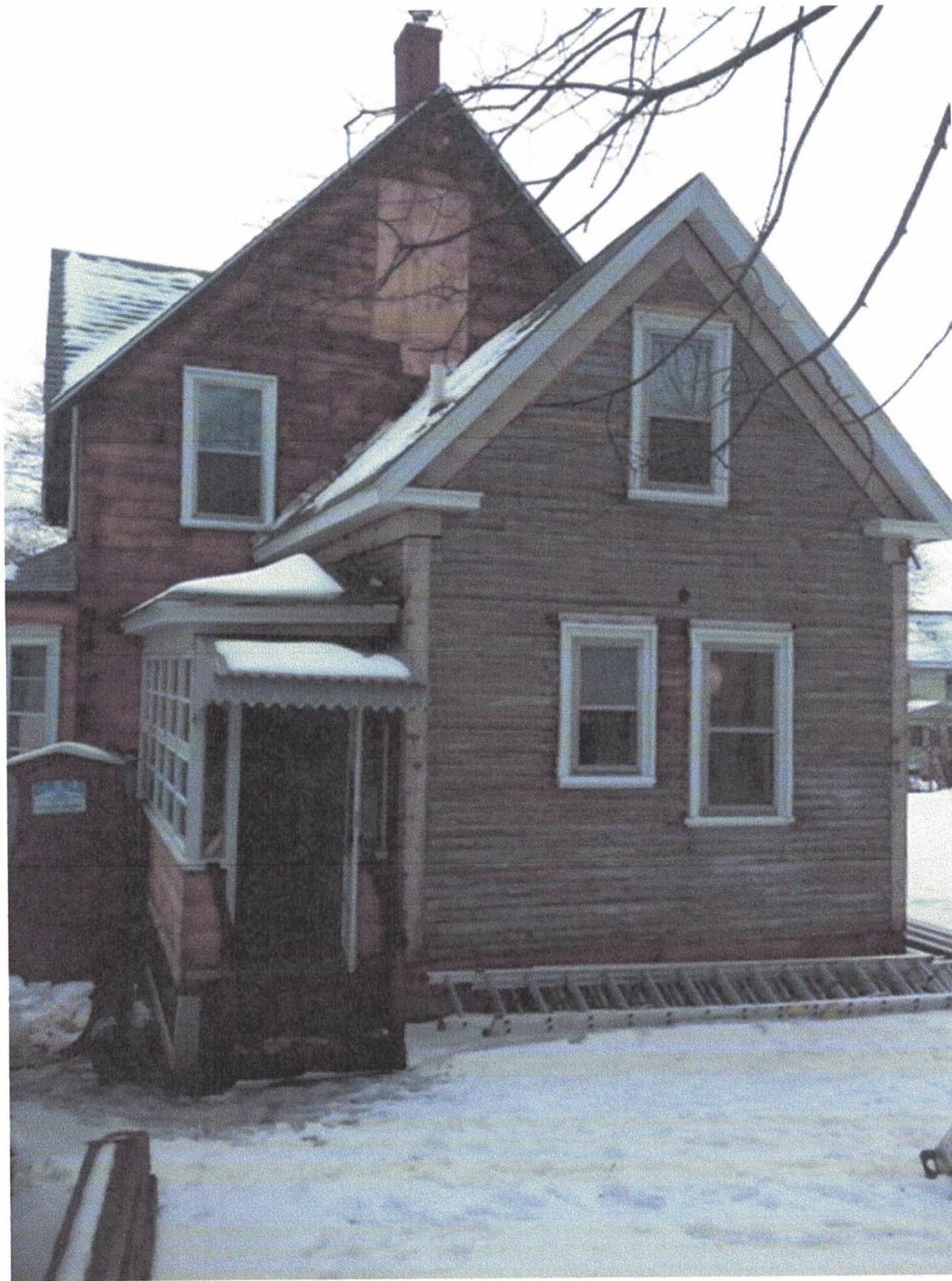
Rear of Existing House
