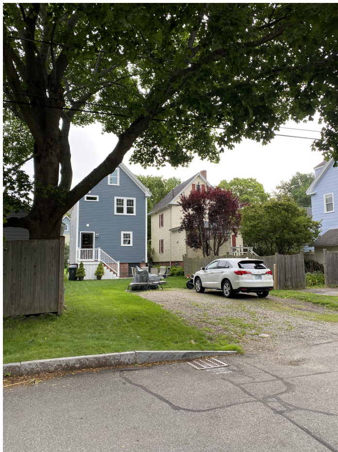
SITE FROM SHERBURNE AVE
