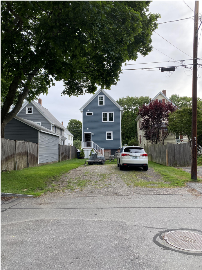
SITE FROM SHERBURNE AVE
